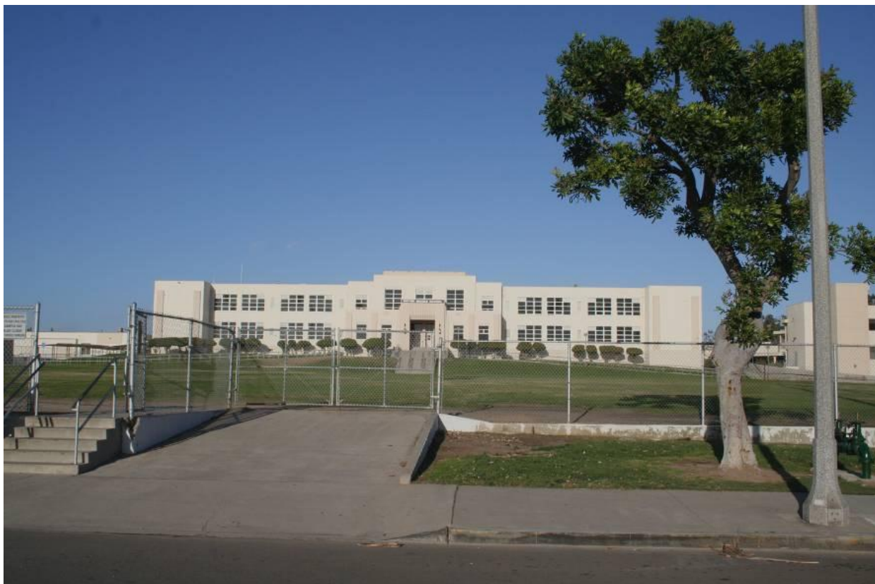
Figure 57: View looking east from Palm at Dwyer Middle School, a good example of Art Deco architecture.
