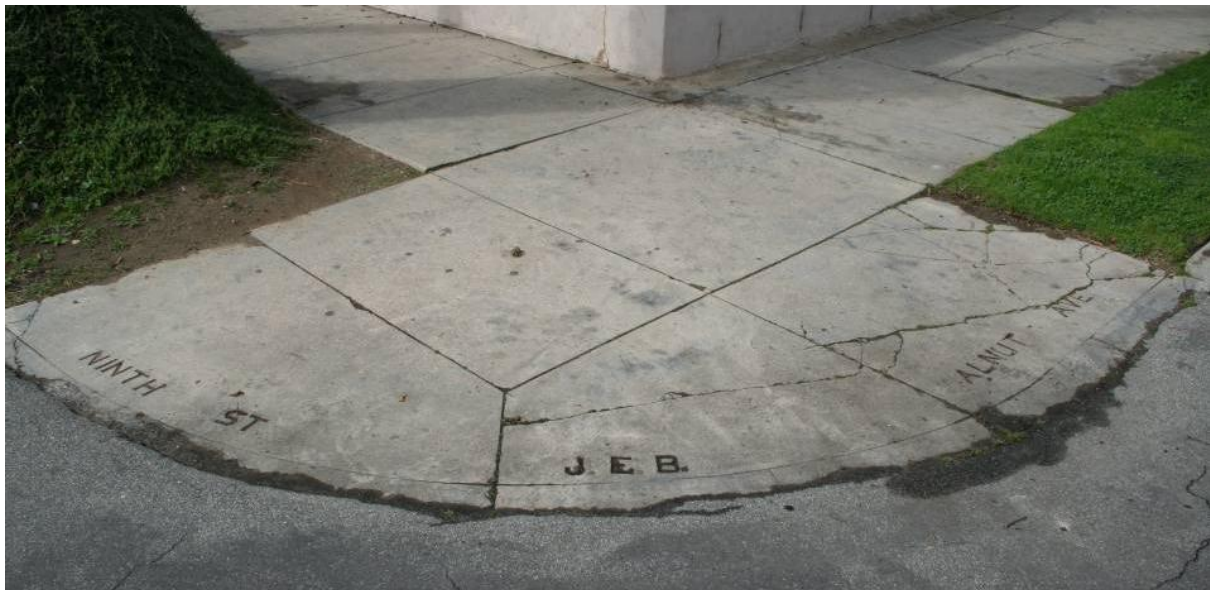
Figure 65: Close-up of typical old concrete sidewalk detail listing the street name "NINTH ST - WALNUT AVE" and the contractor "JEB."
