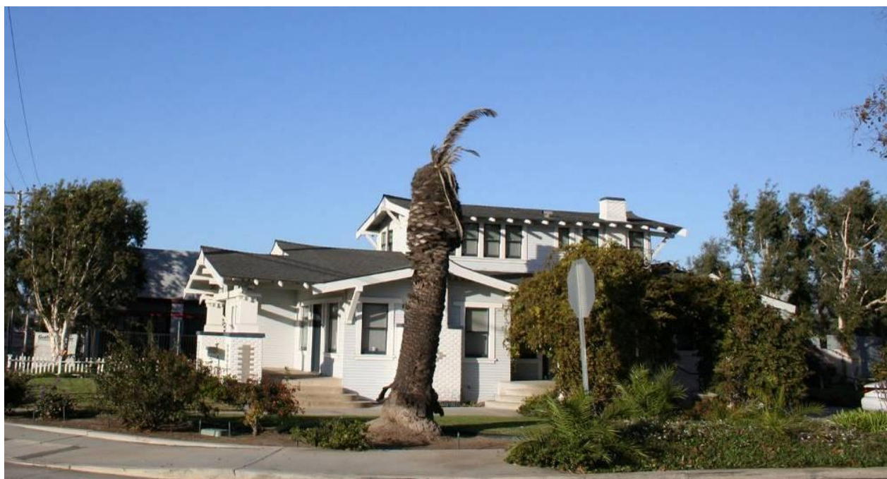
Figure 49: Another example of Bungalow architecture with an “airplane” style second-story atop the building’s complex roof. This example, once owned by the Slater family, is located on the corner of Gothard Street and Cedar Street, the location of Wintersburg.
