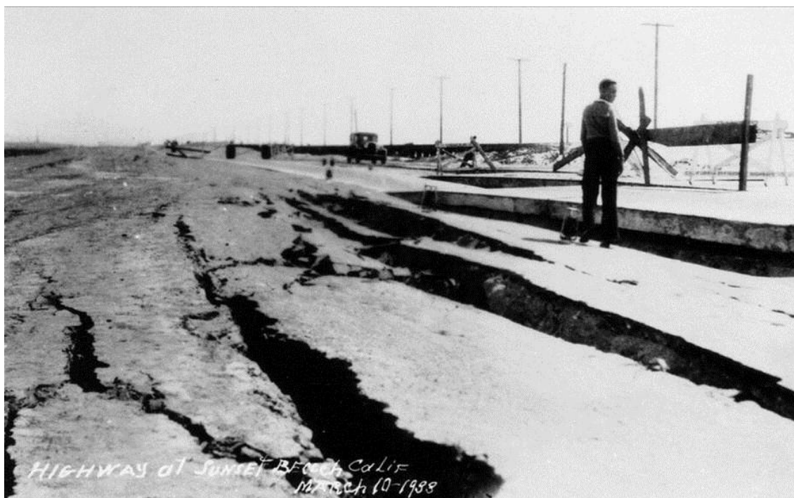
Figure 3: View of damage along the Pacific Coast Highway caused by the Long Beach Earthquake of 1933. Despite its name, the epicenter of the earthquake was beneath the oilfields of eastern Huntington Beach. Photo courtesy of Loyola Marymount University Library, Department of Archives and Special Collections.
