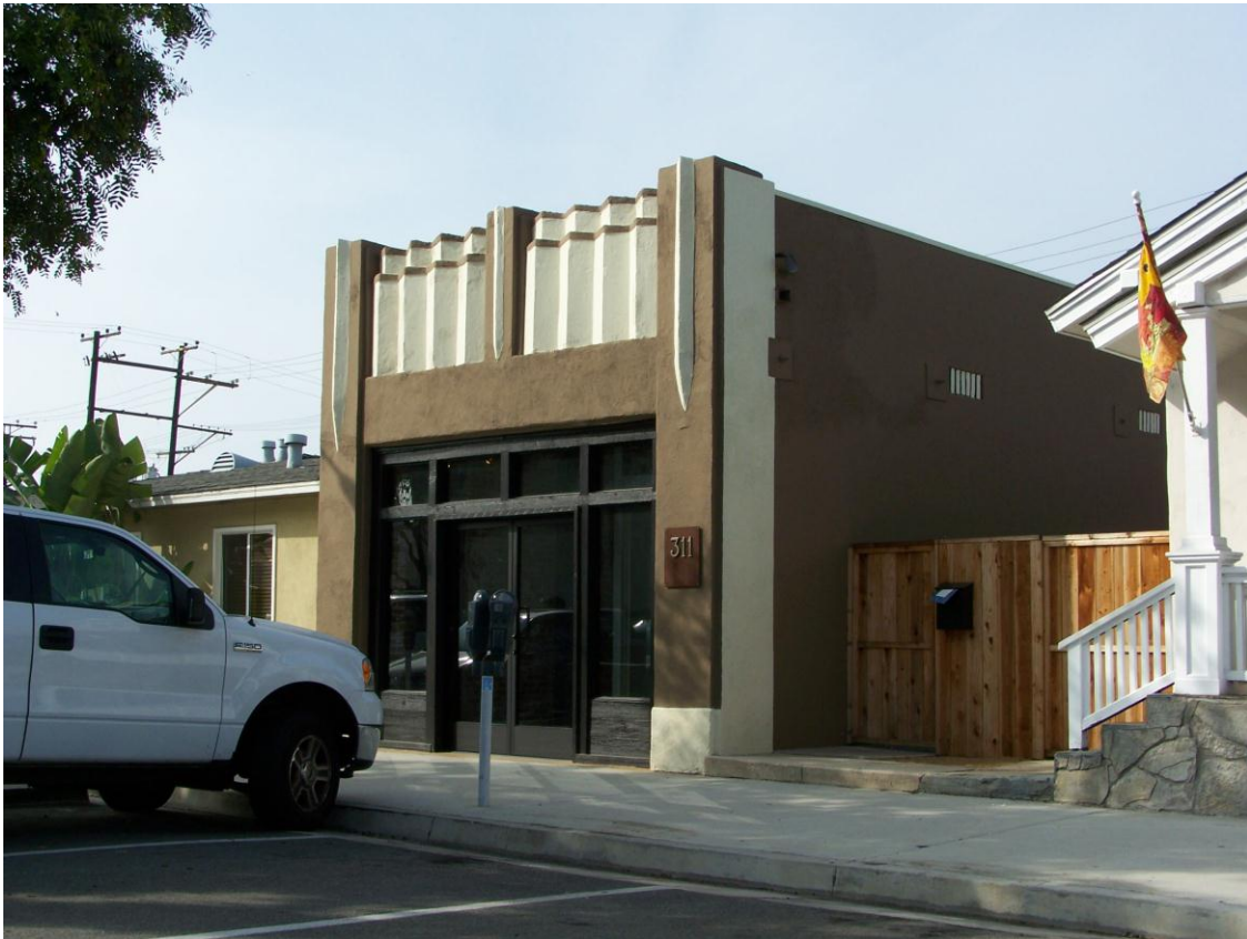
Figure 58: View of 311 5th Street- Zig Zag Moderne commercial building in downtown.
