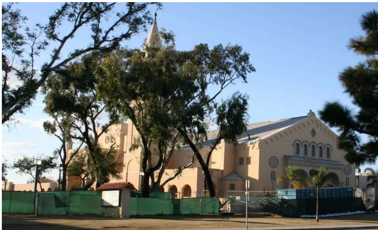
Figure 55: View looking north at Huntington Beach High School from Main Street. The school is listed on the National Register and is designed in the Spanish Colonial Revival style of architecture.
