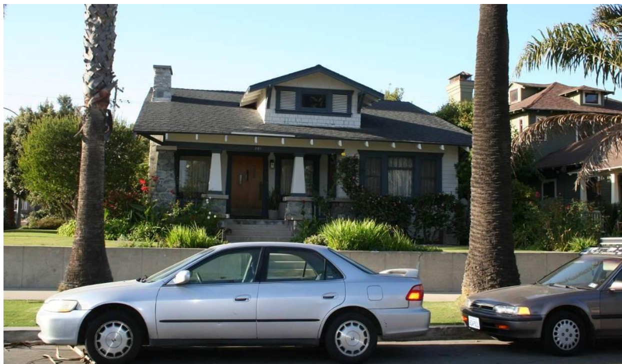
Figure 48: One of the better examples of a true Craftsman or Craftsman Bungalow design, this house is located at the corner of 9 th and Walnut Streets. Note the exaggerated roof, exposed rafter tails, truncated porch columns, half stone and concrete pillar base stone fireplace, and Craftsman windows.
