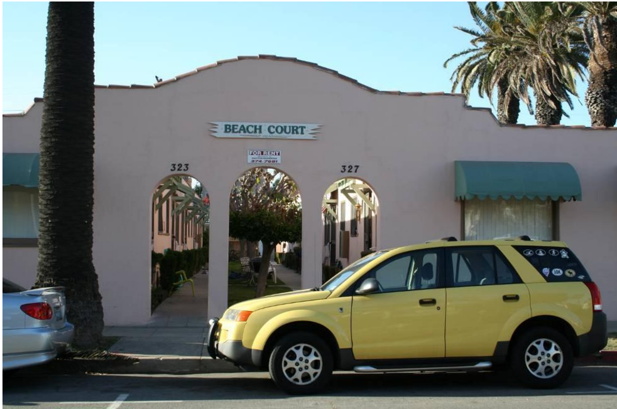
Figure 56: A fine example of a Mediterranean style Bungalow Court, known as “Beach Court,” located at 323-327 6 th Street.
