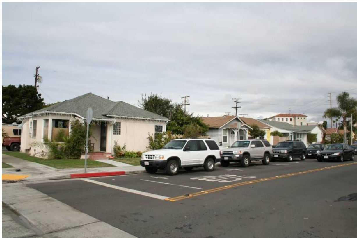
Figure 51: Row of modest cottages from the oil boom years of the 1920s through the late 1930s along Lake Street.
