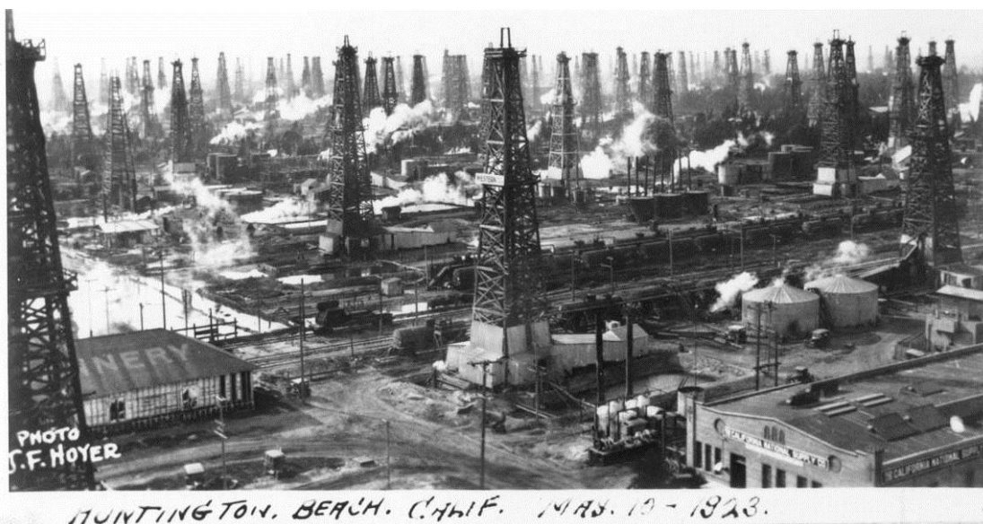
Figure 22: View of Huntington Beach oil fields 1923. The masonry building on the right was owned by the California National Supply Company and the wood-frame building on the left appears to be storage or warehouse shed for the railroad siding. Note the rows of oil tank cars along the tracks and the wooden oil derricks. Courtesy City of Huntington Beach, Centennial Photo Gallery, 2009.
