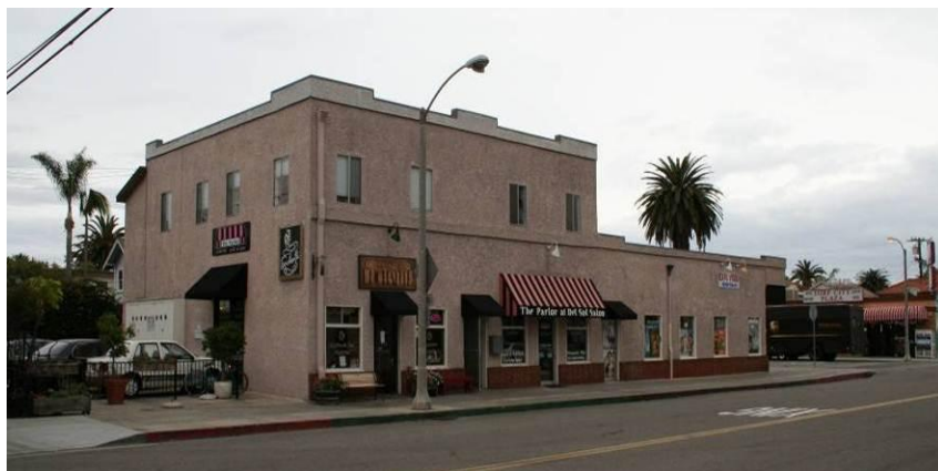
Figure 45: Howard's Market, extensively remodeled and located at the corner of Orange and 11 th Streets.
