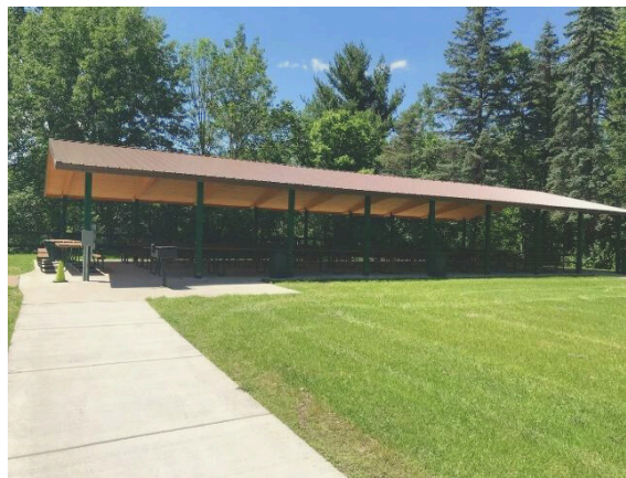
Overlook Shelter Capacity: 240 people
