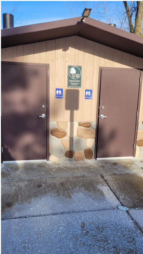
Photo G. Trust Fund plaque located on the restroom building.
