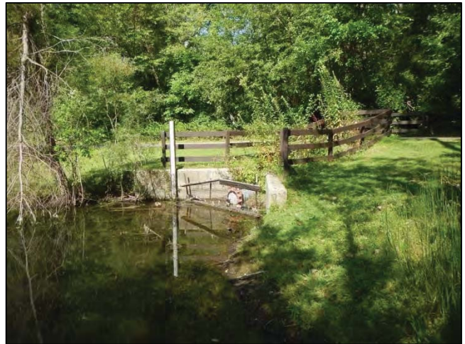
Photo 116: Culvert & headwall for overflow at Lake
