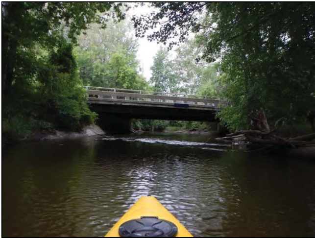
Photo 2: Looking west at N. Aurelius Rd.
