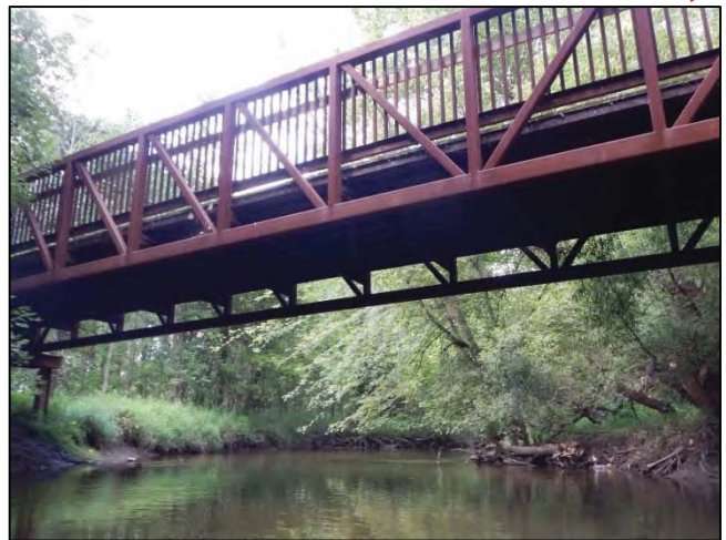
Photo 32: Looking north at the Lansing River Trail
