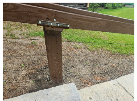
Wire Railing Install
