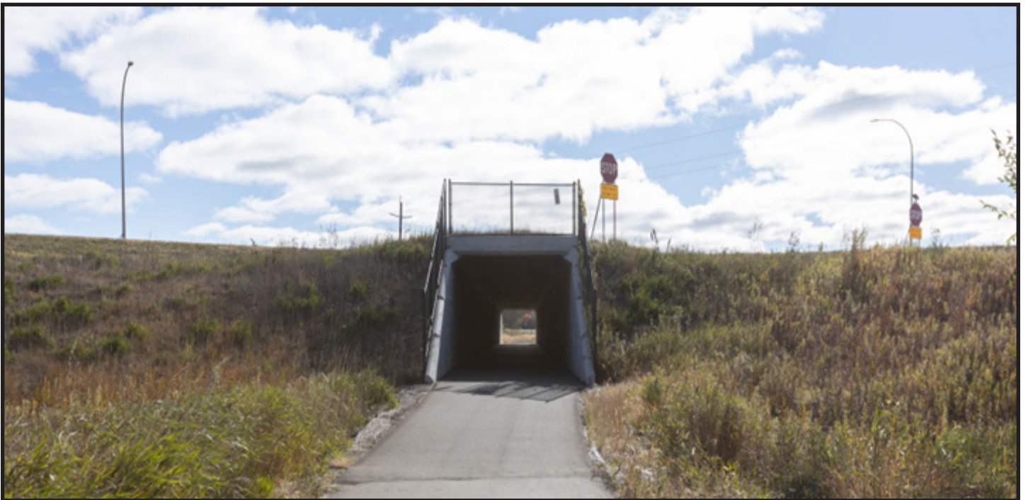
A pedestrian underpass allows trail users to cross U.S. Hwy. 71 and Kandiyohi County Rd. 40 without traffic
