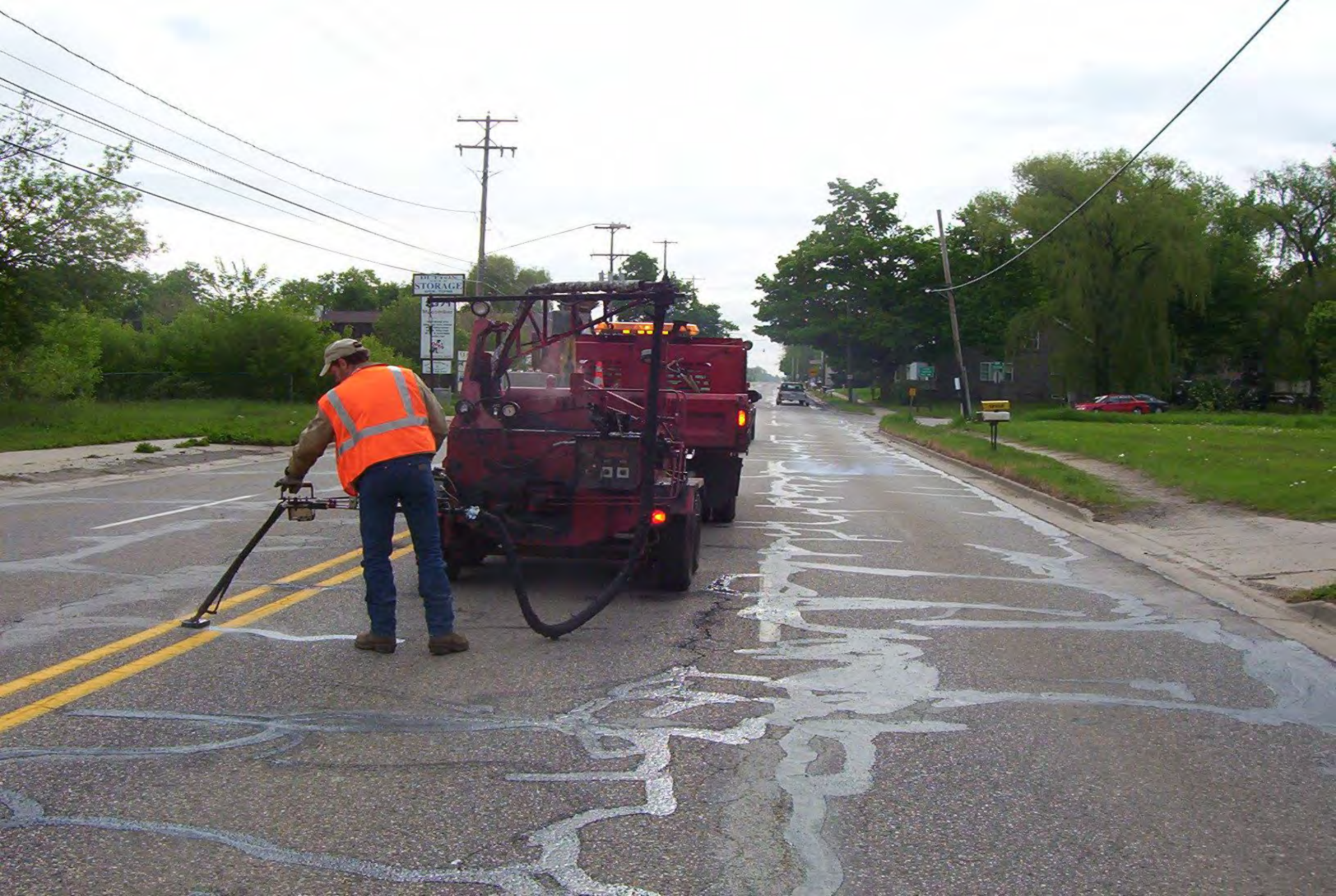
Crack Sealing
