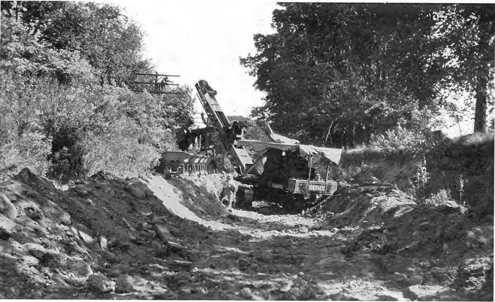
Making a cut with gasoline shovel and industrial railway in the hill just east of the Cascade Bridge on M-16.
