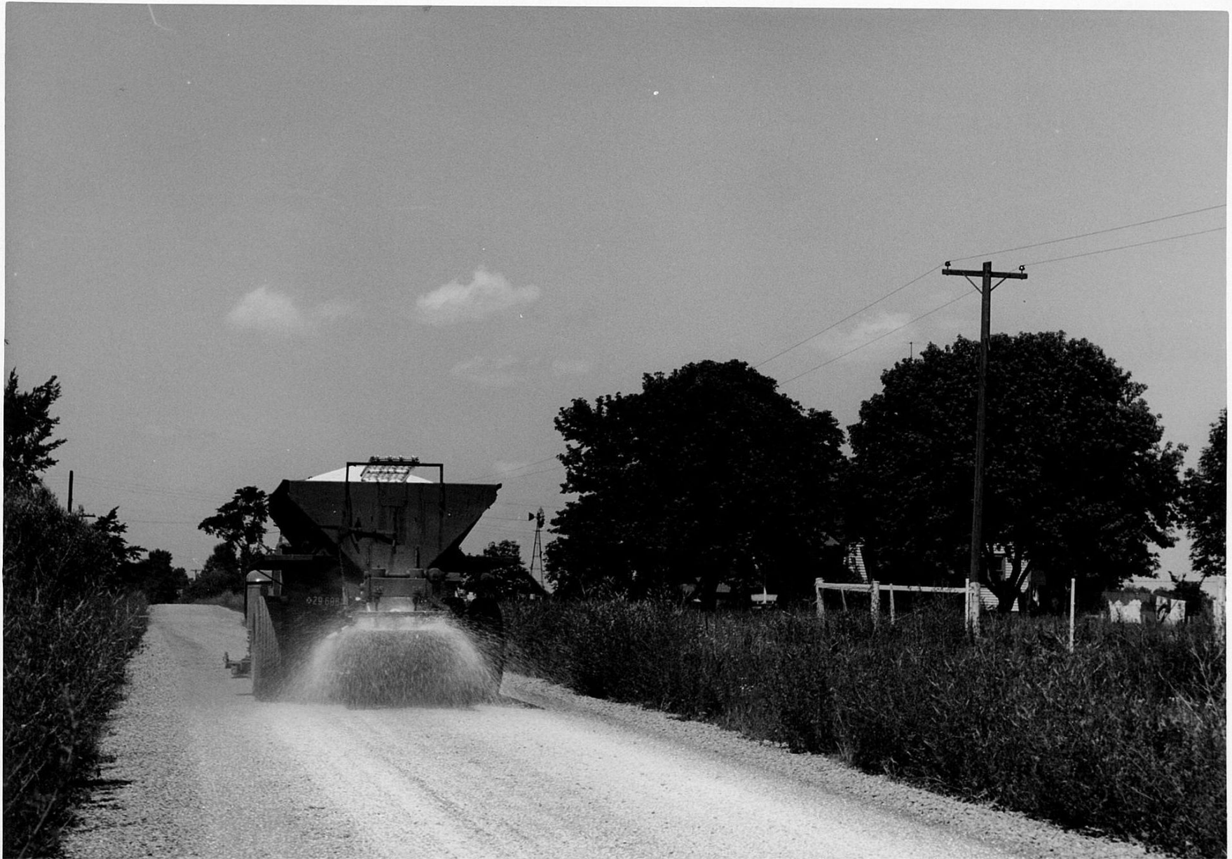
Spreading Chloride
