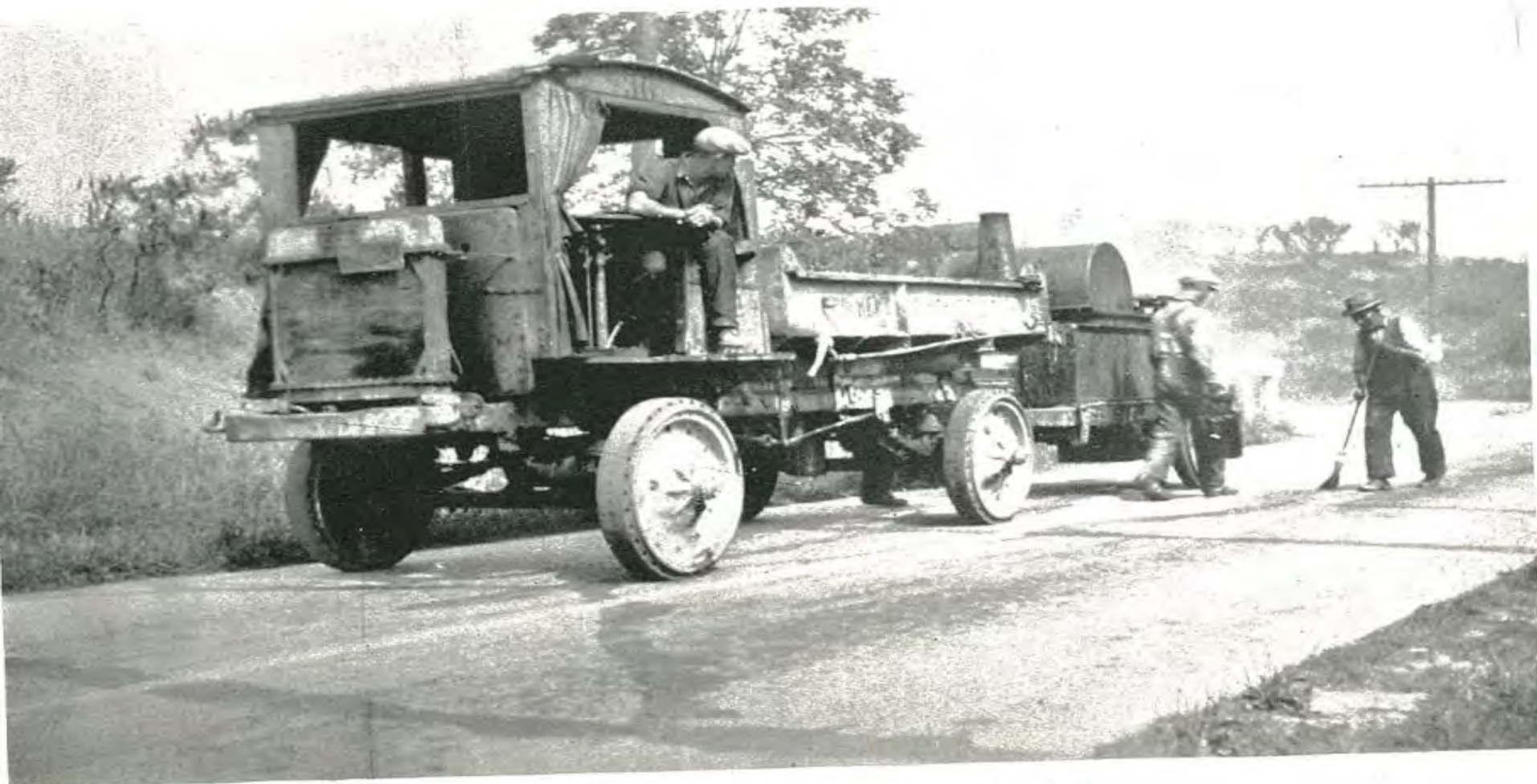
Tarring Cracks and Joints on a Concrete Road
