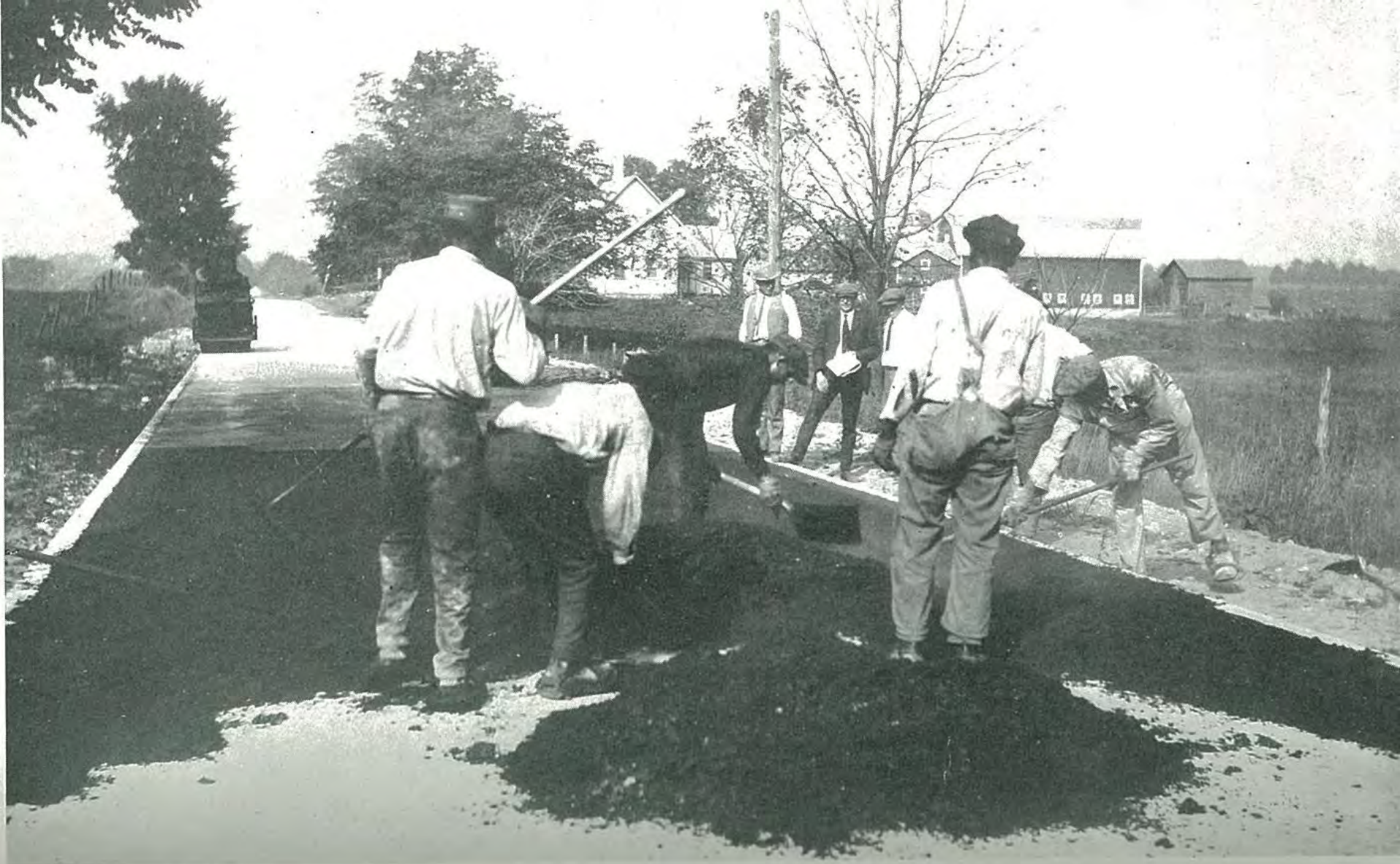
Laying 2-inch Asphalt Top (Topeka mix) on T. L. No. 54 North of Sparta
