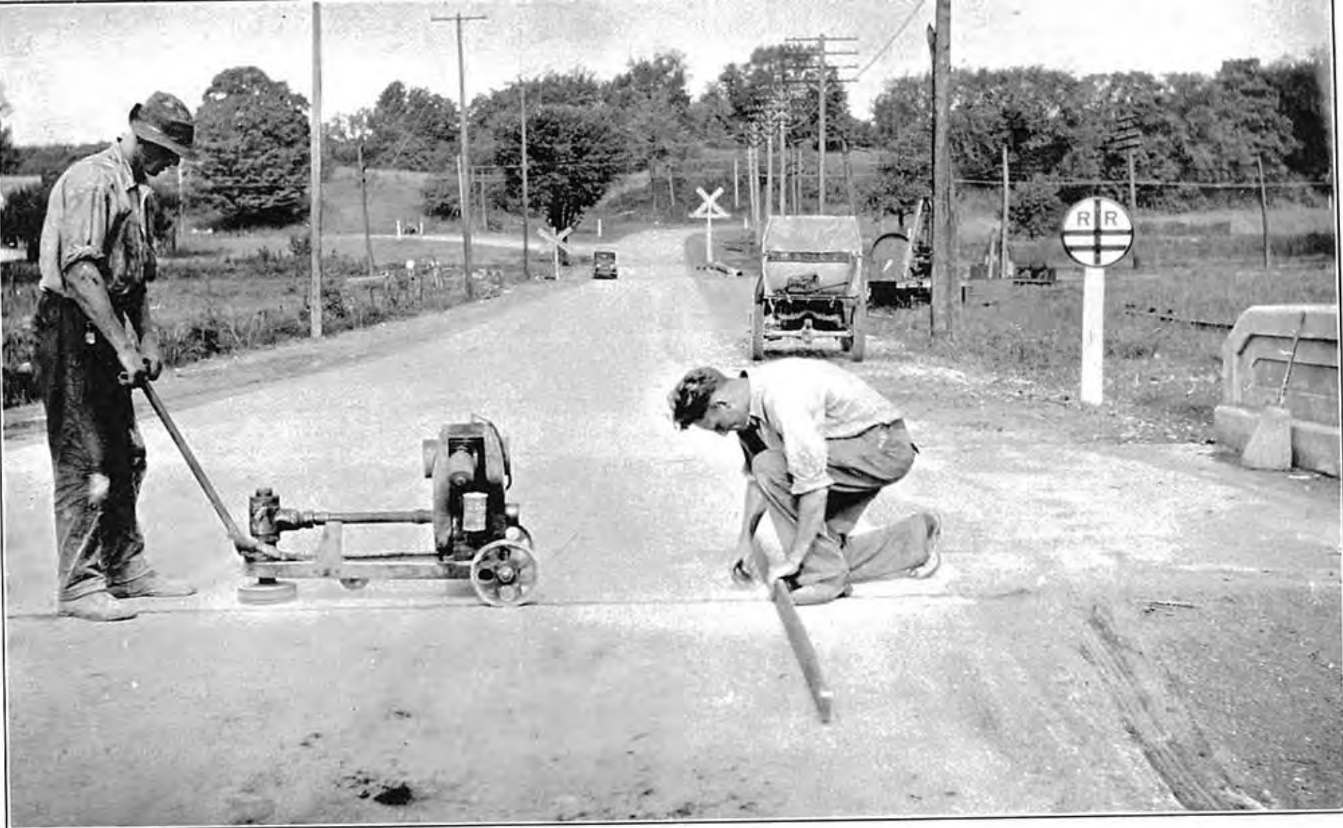
Grinding down high spots on a new concrete pavement.
