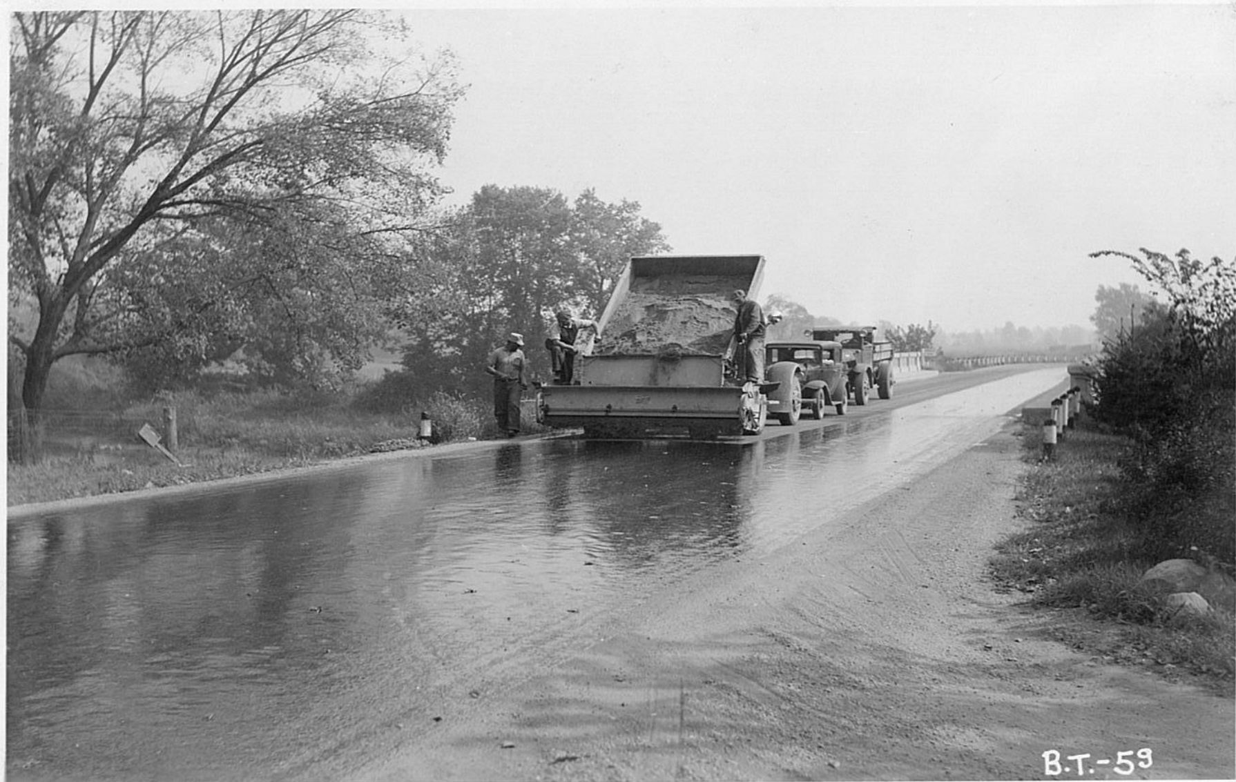
Spreading Stone
