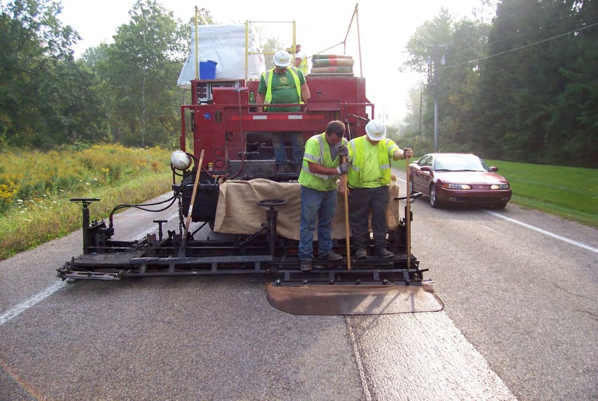
Slurry Seal
