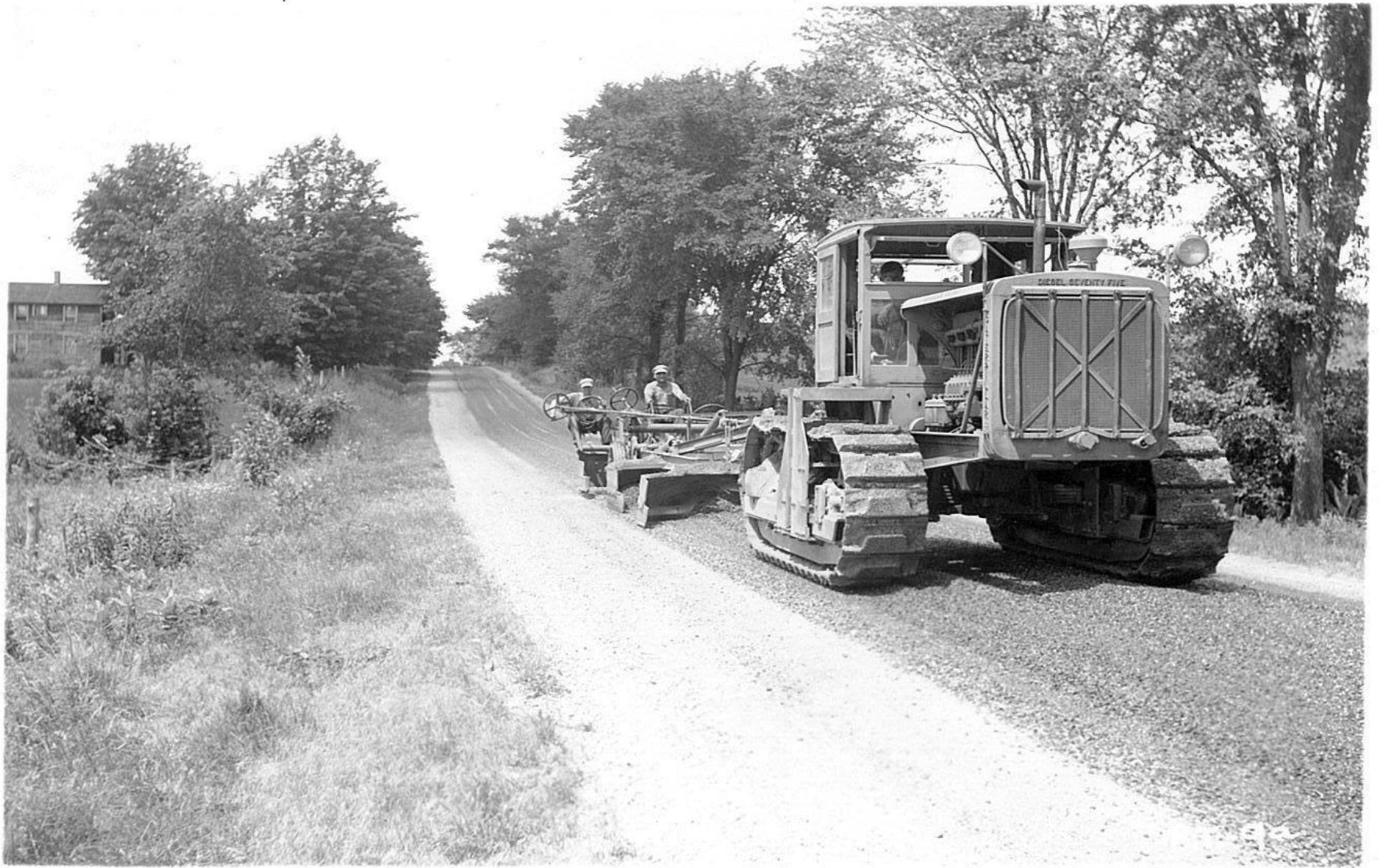
Grading cold mixture
