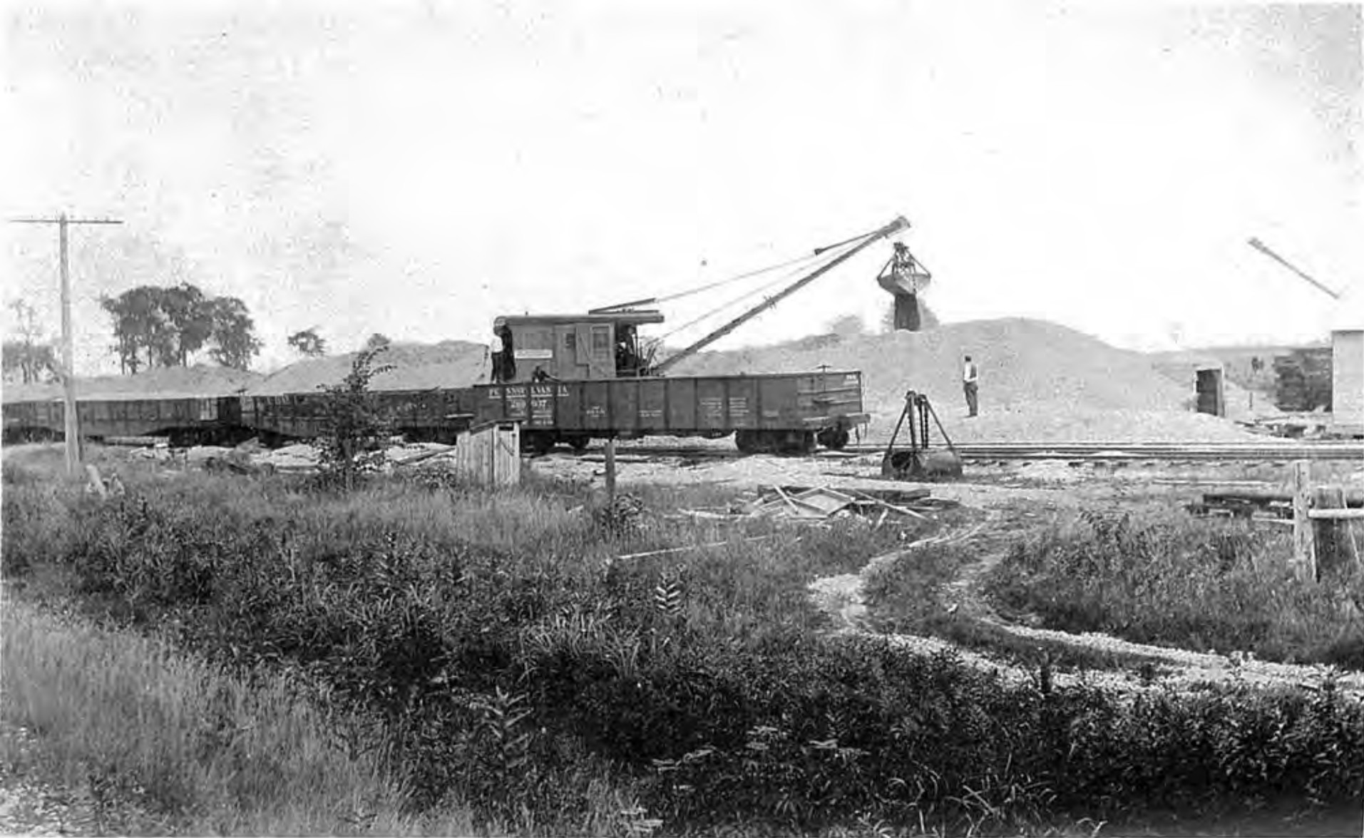
Unloading gravel and sand and placing over tunnel at Carlisle.
