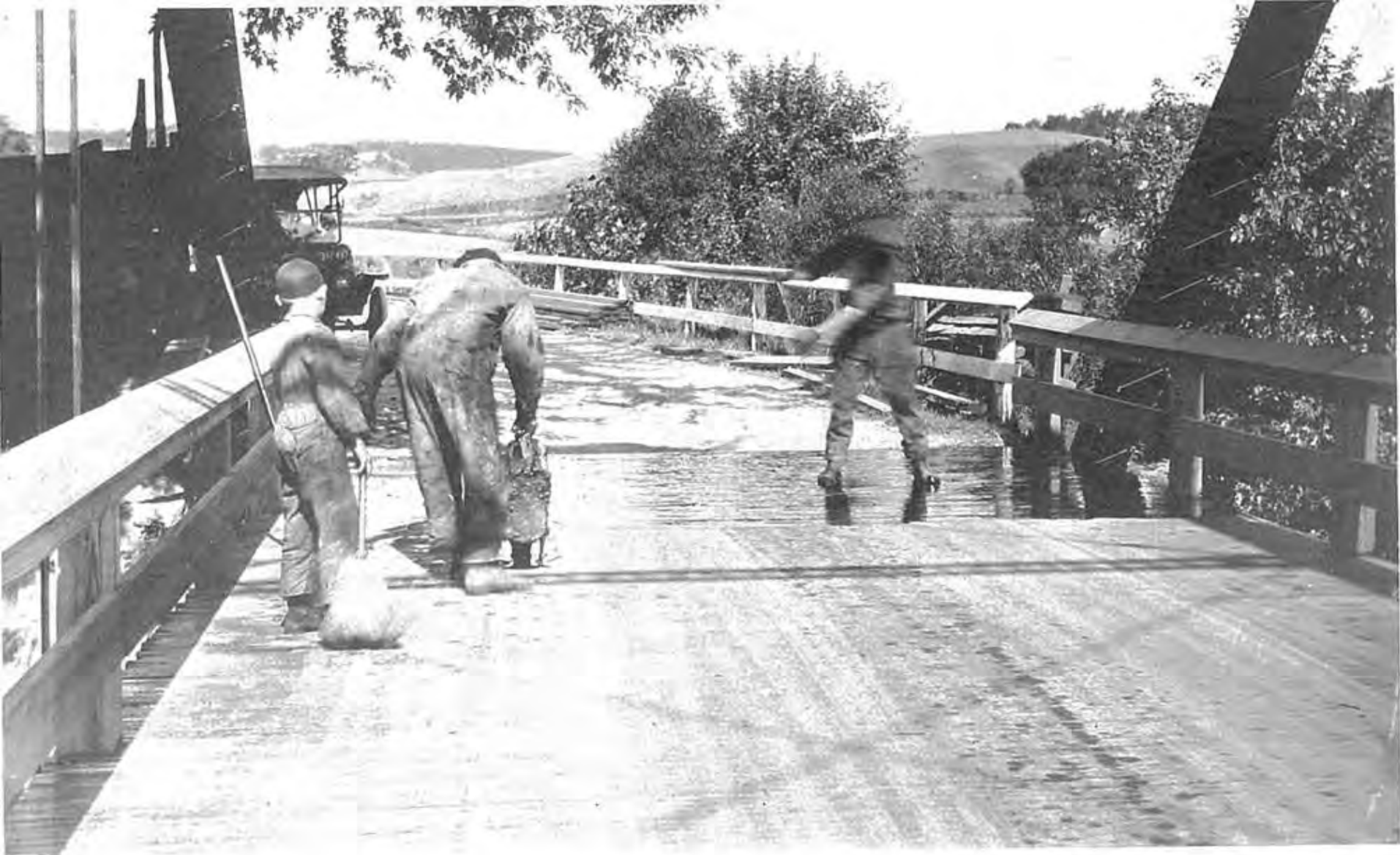
Knapp Bridge—placing seal coat of tar on new floor to waterproof the surface.
