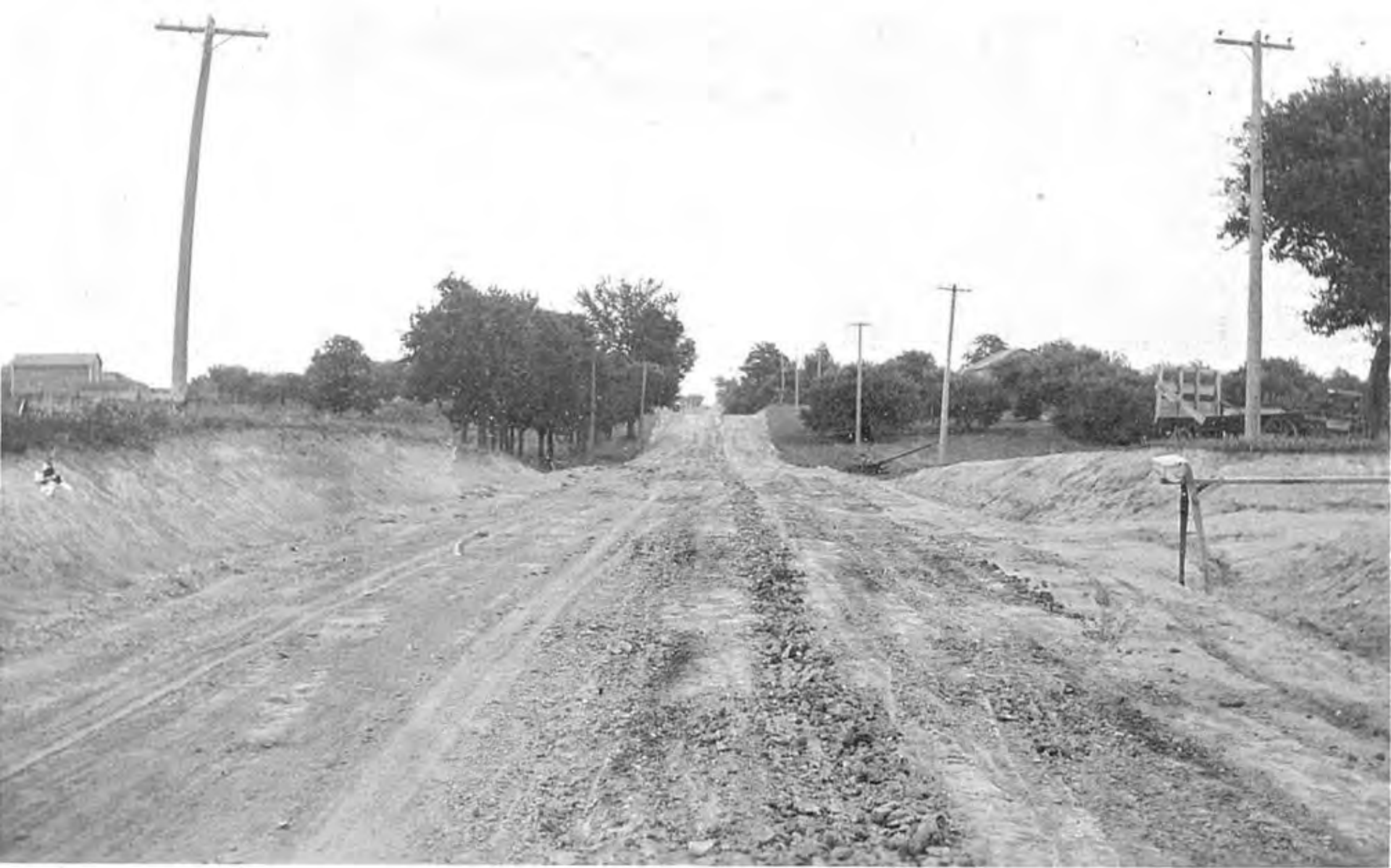
Cedar Springs-Solon Road showing flat earthgrade. First step in the construction of a gravel road.
