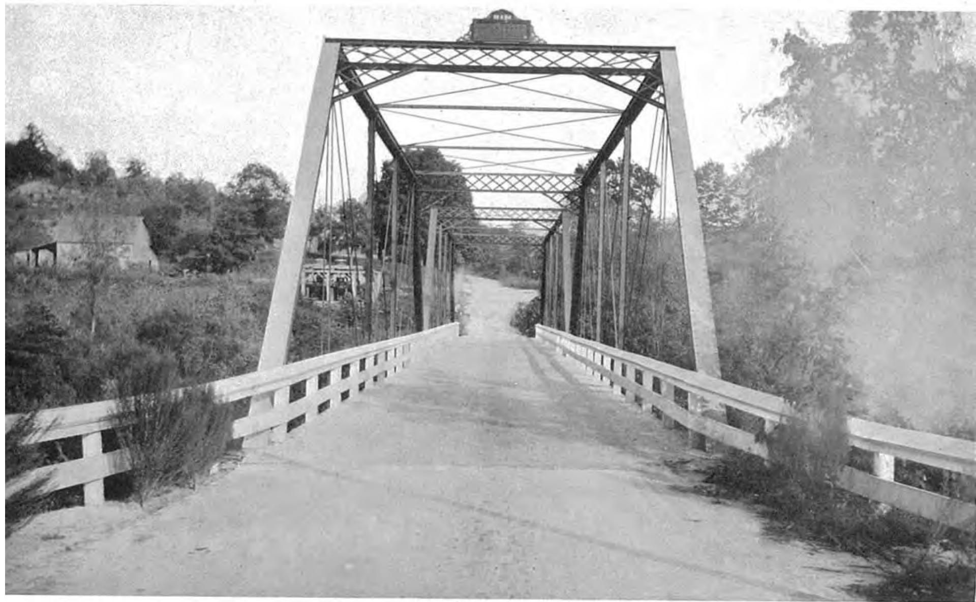
The Alaska Bridge which has been given a new floor, two coats of paint and a new guard rail.
