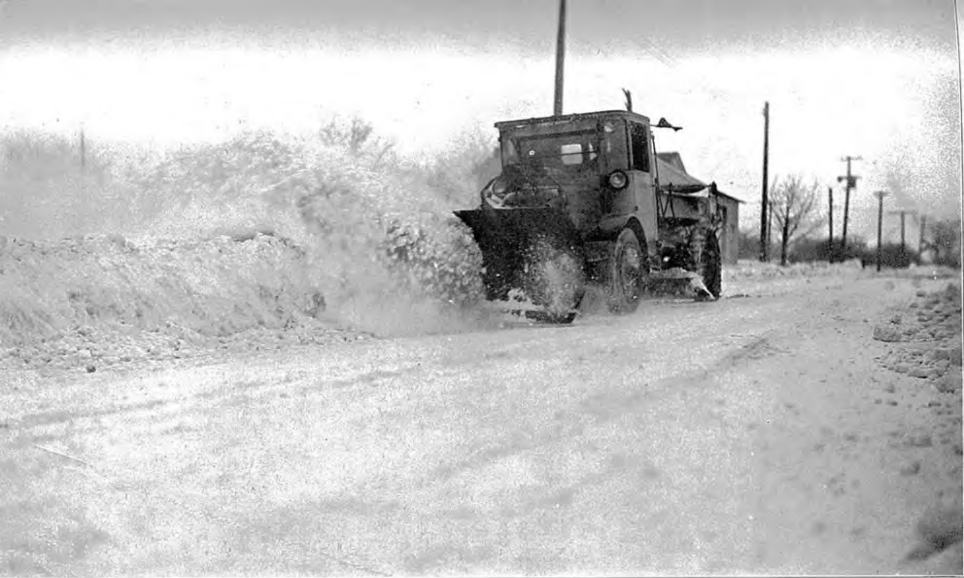
Clearing the roads for action. This powerful truck equipped with a blade plow makes short work of drifts and snow windrows such as the one shown here.
