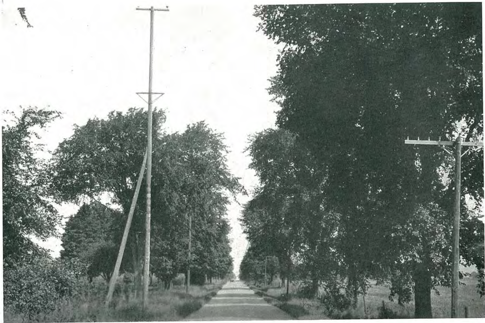
On the Walker Road near Kent City showing high and low pole lines placed so as to avoid trimming and mutilating trees. This work is controlled by our Forester.
