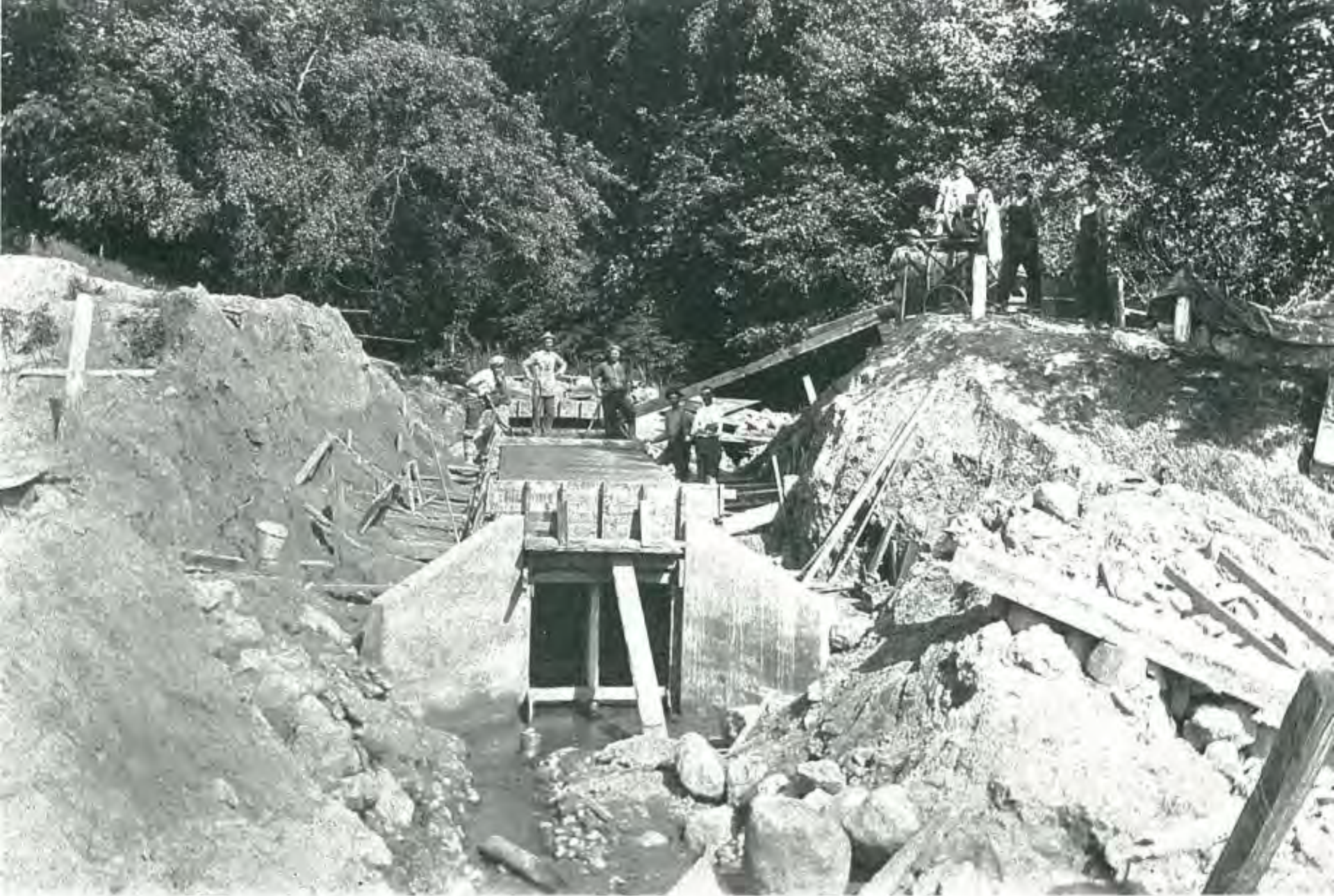
A typical reinforced concrete box culvert under construction on M-13 south of Grand Rapids.
