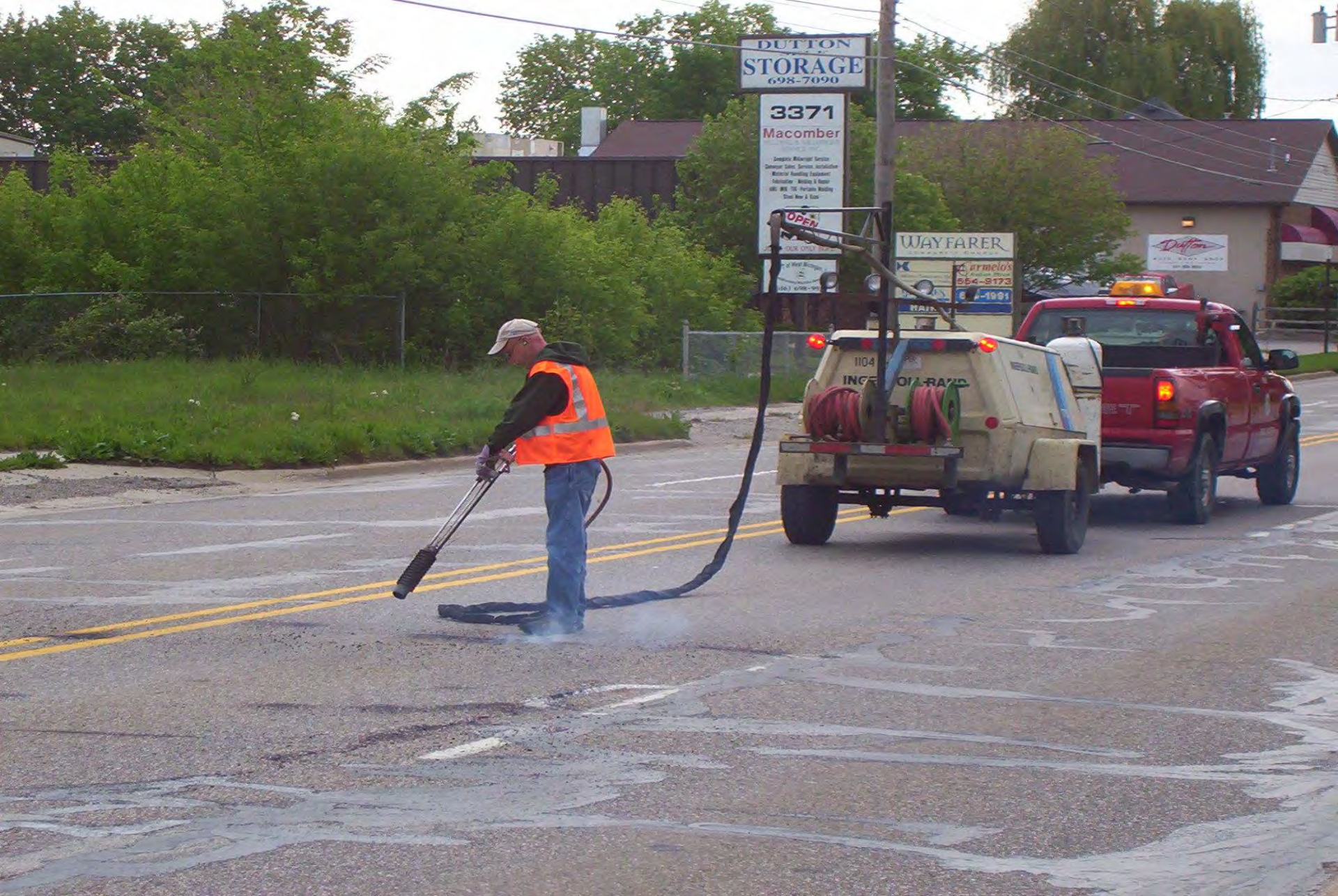
Crack Cleaning
