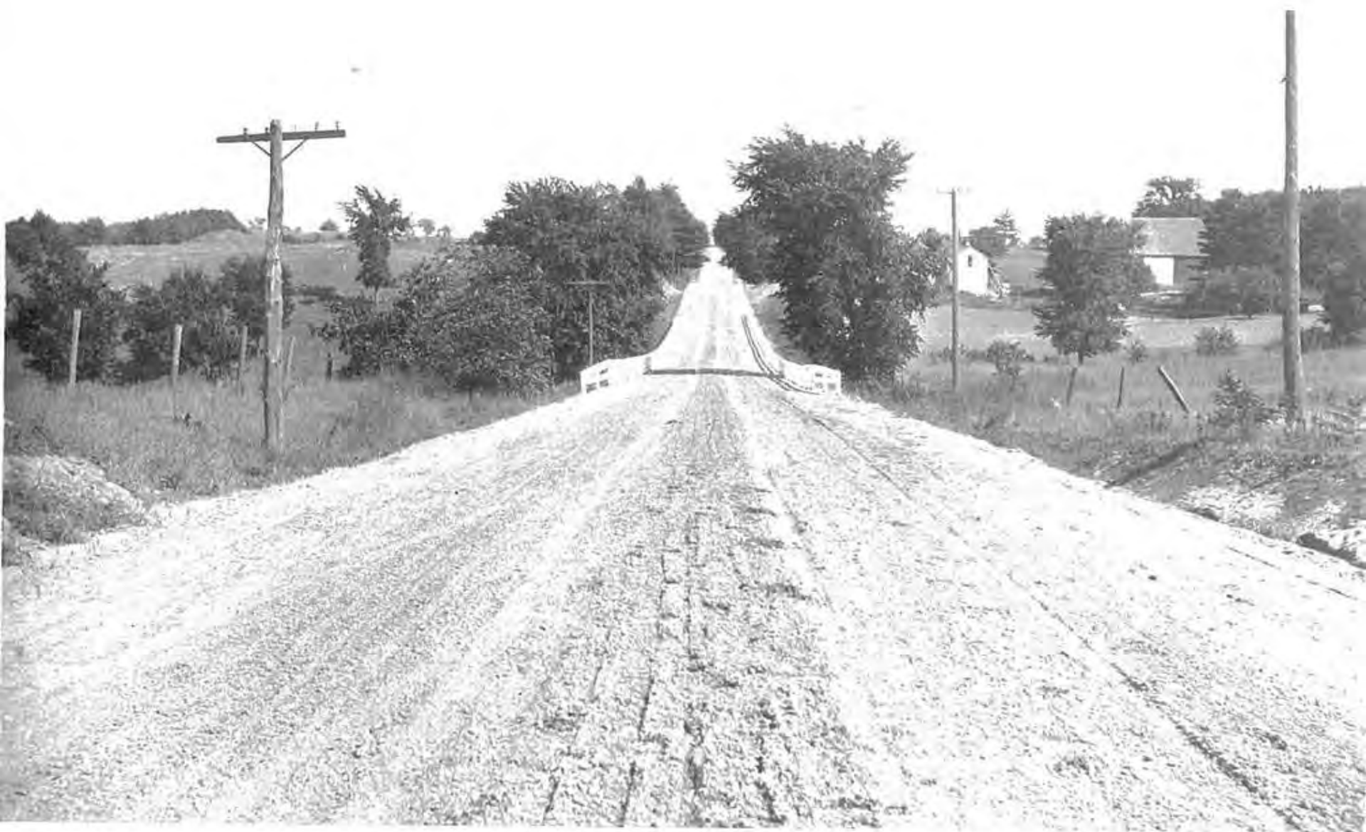
Looking East on the Cedar Springs-Solon Road just after the top course of gravel had been placed and the grade trimmed.
