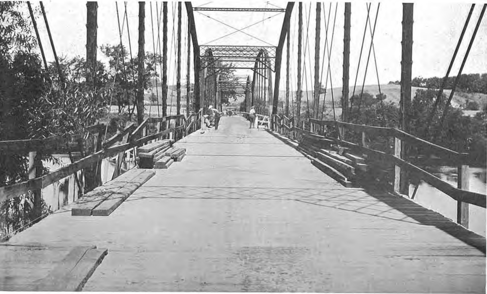
Placing new floor and guard rail on the Knapp Bridge over Grand River. Traffic was not interrupted while this work was being done.
