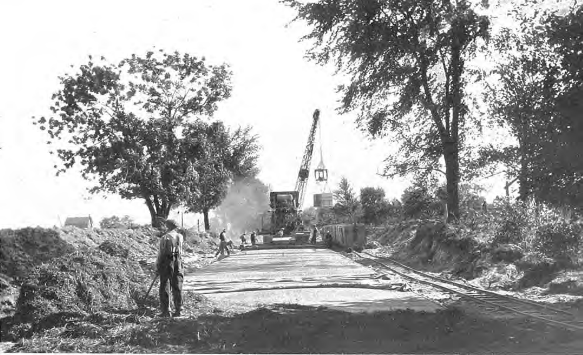
Laying concrete on the new route of M-39 northeast of Alto.
