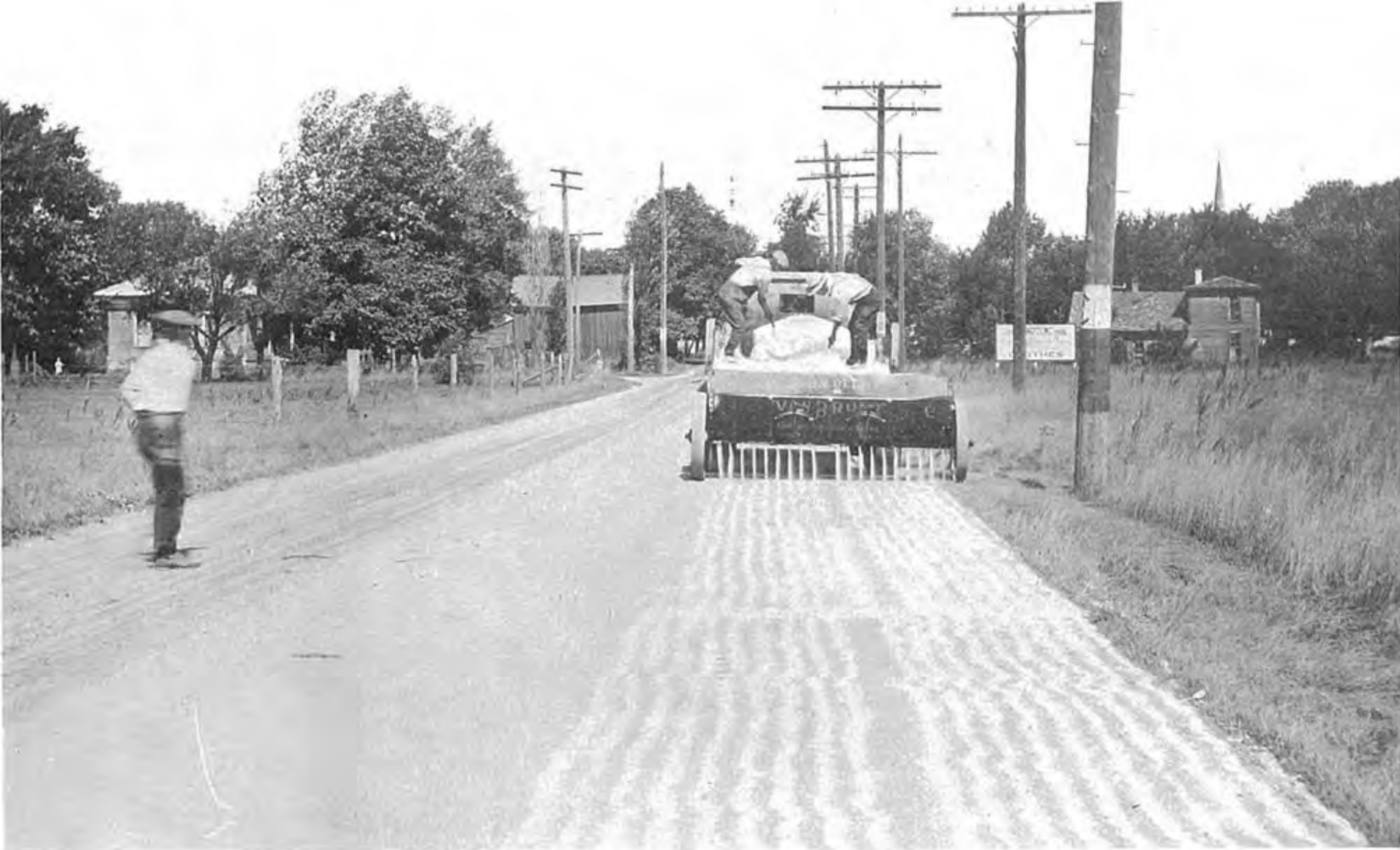
Spreading Calcium Chloride to lay the dust on T. L. No. 16 just East of Lowell.
