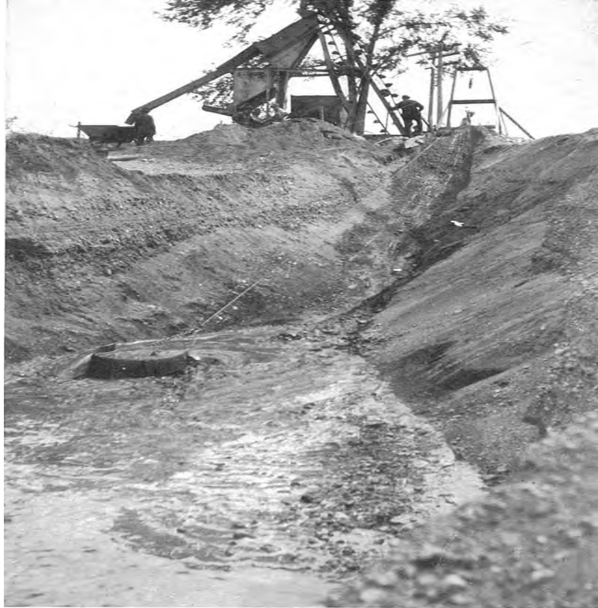
One of our portable screening plants operating in a pit on the Canal Road. This shows how we get gravel out of a bad place.
