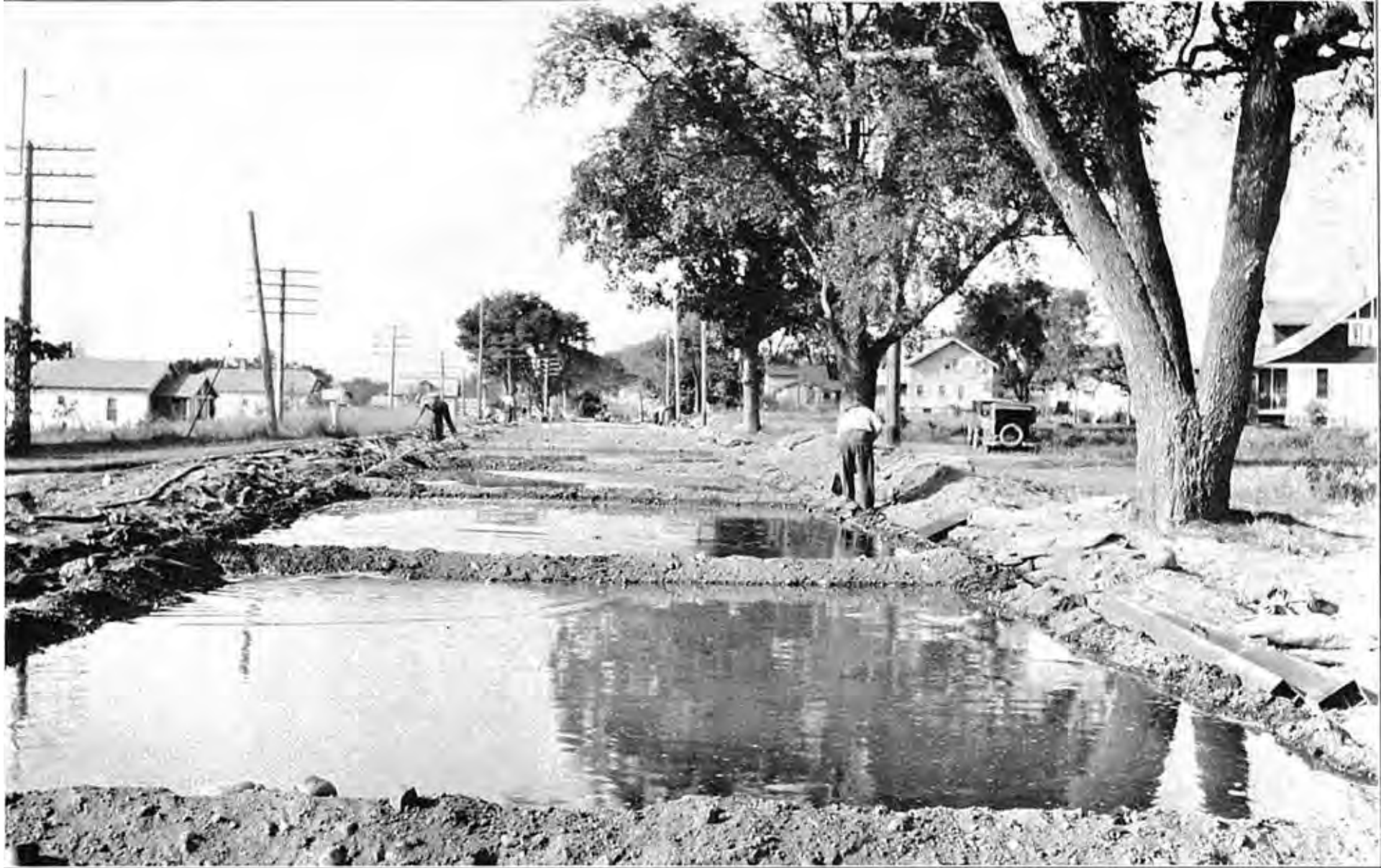
Curing a 20-ft. concrete road by the ponding method—the West River Road near Comstock Park.
