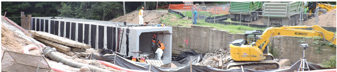
Crew installs new box culvert at Podunk Avenue.
