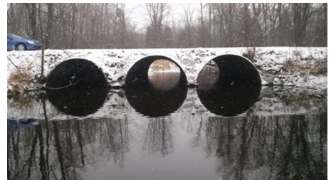
The 108th Street Bridge (top); Three culverts that collectively span more than 20 feet are defined as a bridge (bottom).
