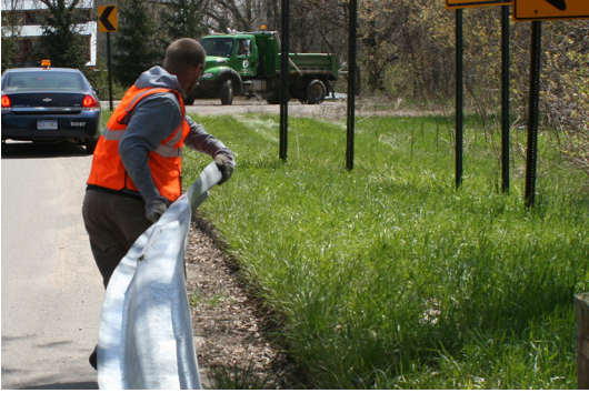
Figure 7 Guardrail Installation
