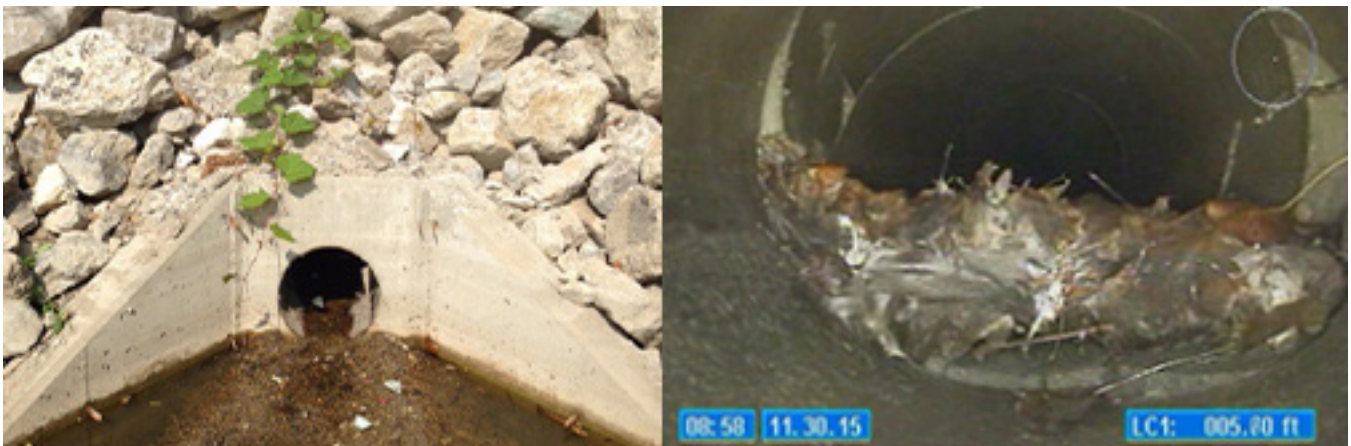
Storm sewer outlet (left); Video still showing debris restricting storm sewer (right)
