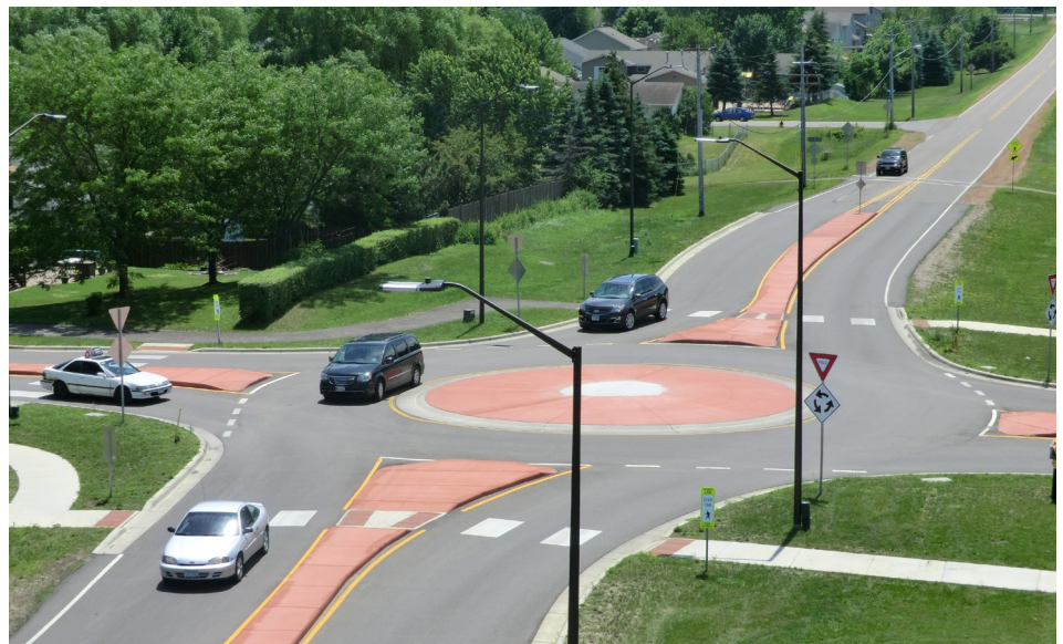
Example of a single-lane roundabout. Source: FHWA
