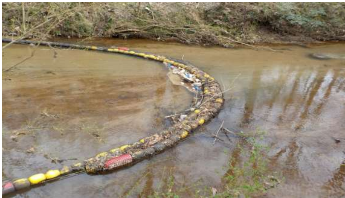
The Trash Trap located on Blue John Creek just upstream of the Orchard Hill Road Crossing. Note the trash that has collected on the trap. Trash is removed on a weekly basis.
