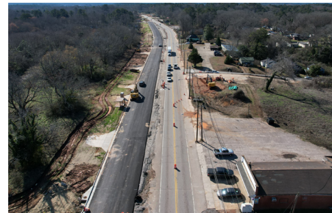
GDOT's Hamilton Road widening project
