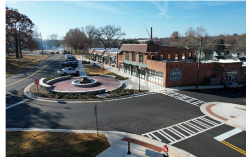
Lincoln Streetscape in the Hillside community
