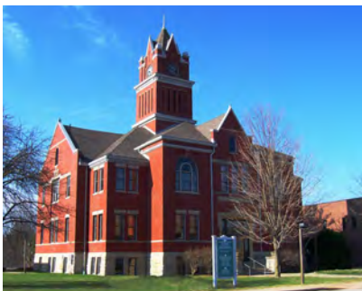
Antrim County Courthouse 203 E. Cayuga St. Bellaire, MI 49615
