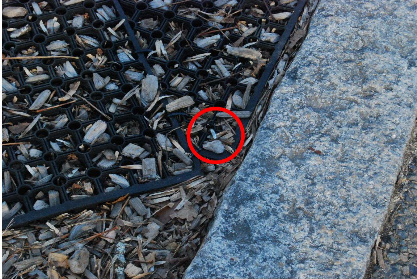
The mats are secured to one another by the regular placement of zip ties to ensure they provide a continuous surface between mats.
