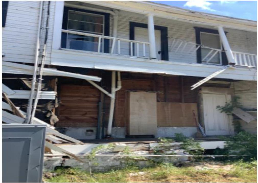
Rotten wood and termite damage on upper rafters:
