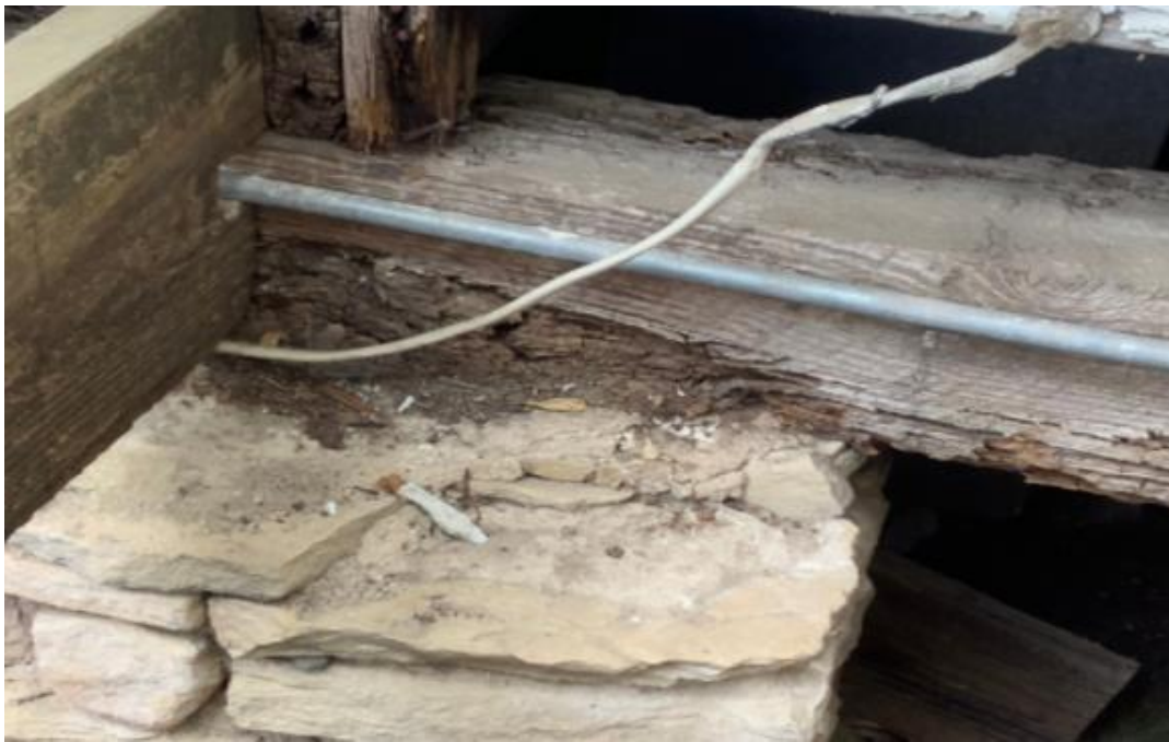
Termite damage on foundation beams. This is the foundation under the East side porch
