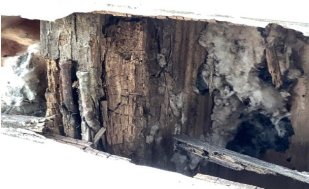
Photo: Rotten studs
