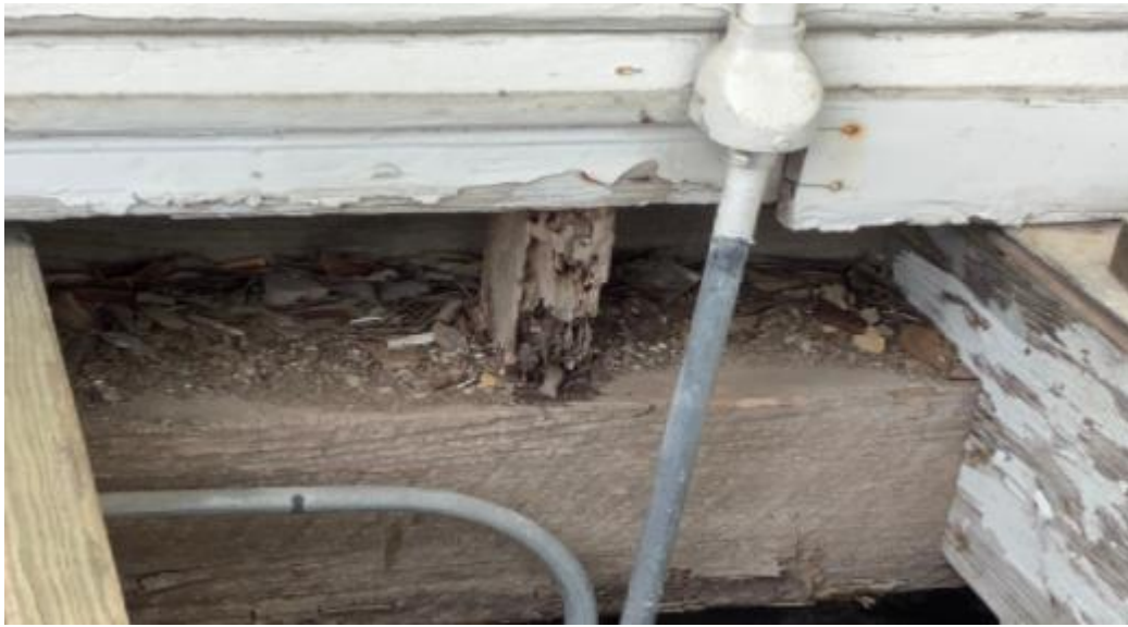
Termite damage on foundation beams. This is the foundation under the East side porch
