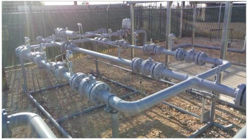
Newly constructed natural gas regulator station and site piping.
