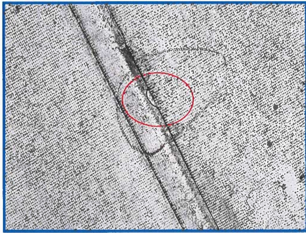
City of Navasota / Rec Center / Hail Exposure Damage / PVC Membrane fracture
