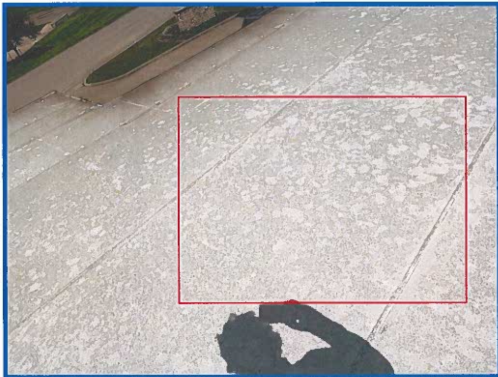
City of Navasota / Rec Center / Hail Exposure Damage / Hail distribution / North Wing
