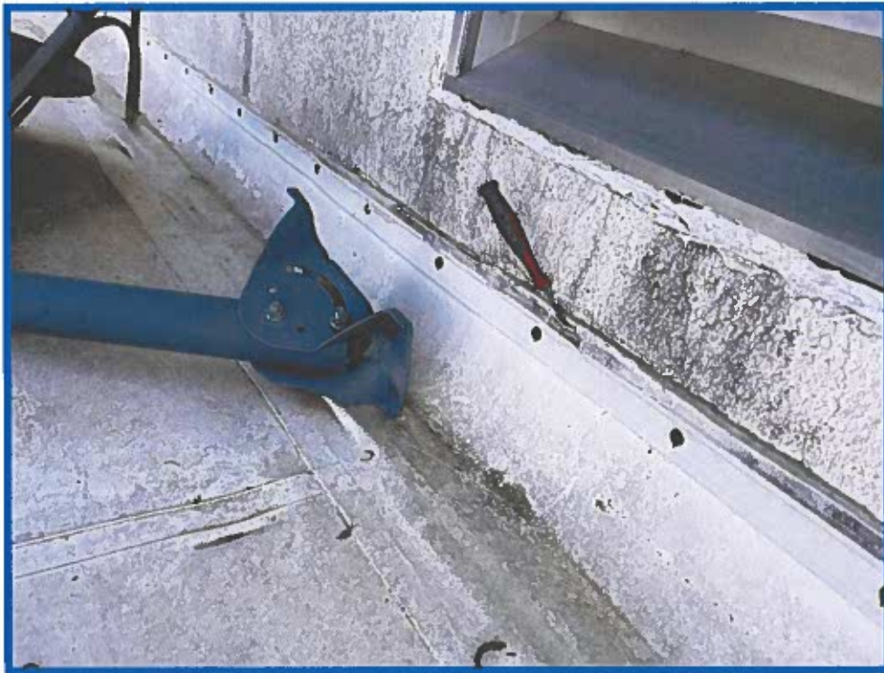
City of Navasota / Rec Center / Wall to deck transition with upper roof / Flashing termination
