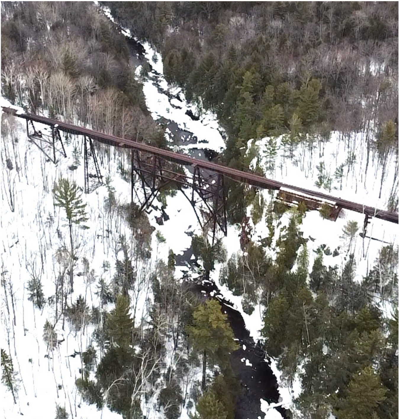
Morgan Creek Rail Trestle
