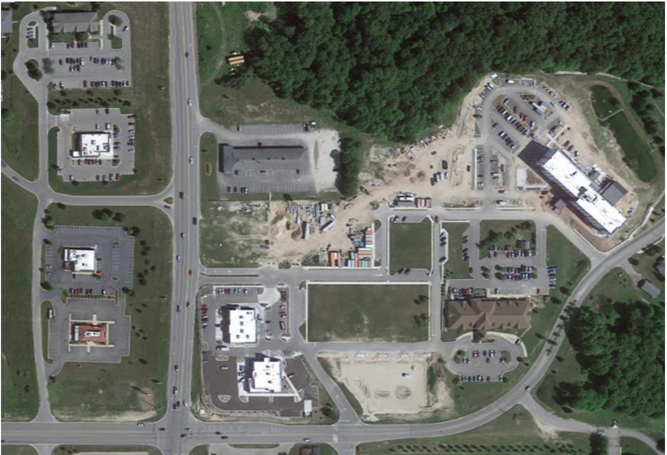
Perpendicular development under construction along US-131 in Bear Creek Township, Emmet County (example reference photo)
