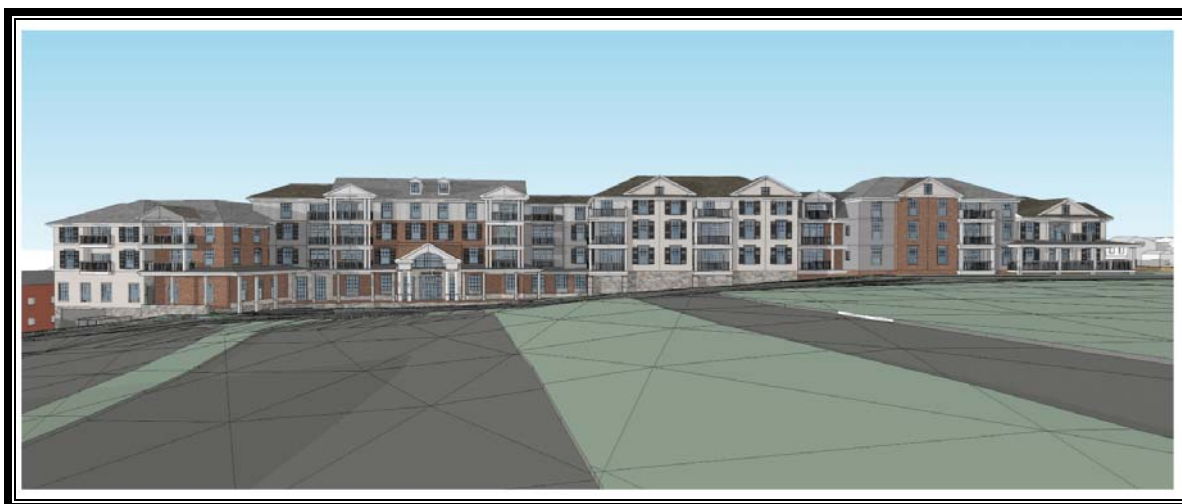
View of North Elevation
