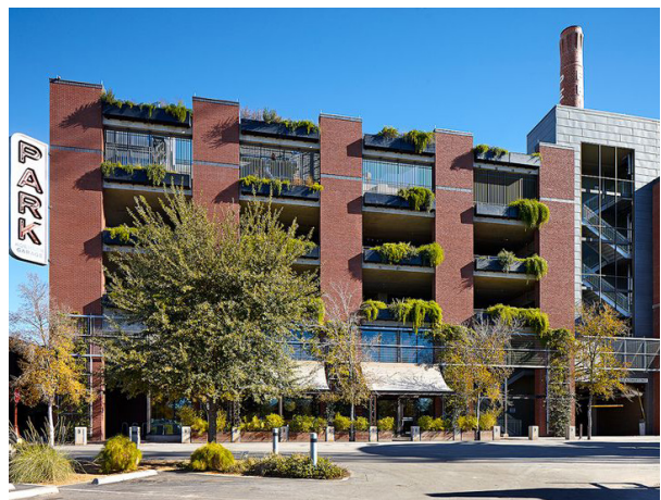
Figure 10. Public Parking Garages
