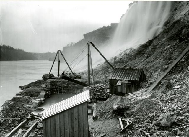
Above: Men using a crane to dredge rocks during construction of Power Station #2, ca. 1896
