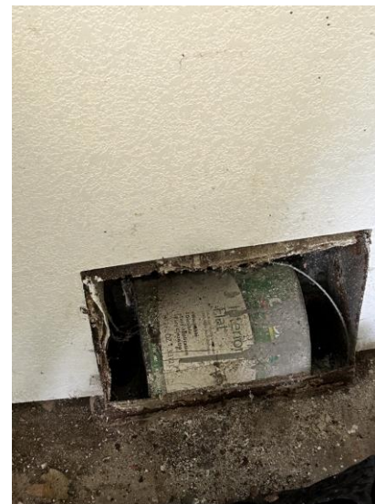
HA #3 typical register with duct wrap
