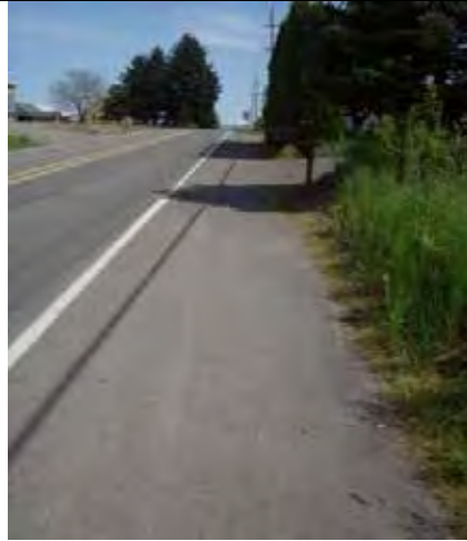
Figure 10: Ideal road shoulder used by pedestrians where bollards, curbs, and/or street reflectors could be installed.
