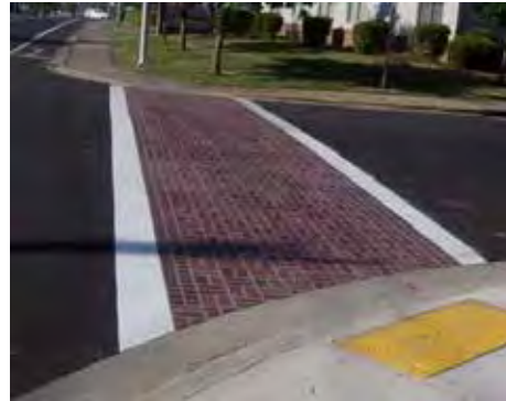
Figure 9: Thermoplastic brick crosswalk, Cottage @ Glencoe
