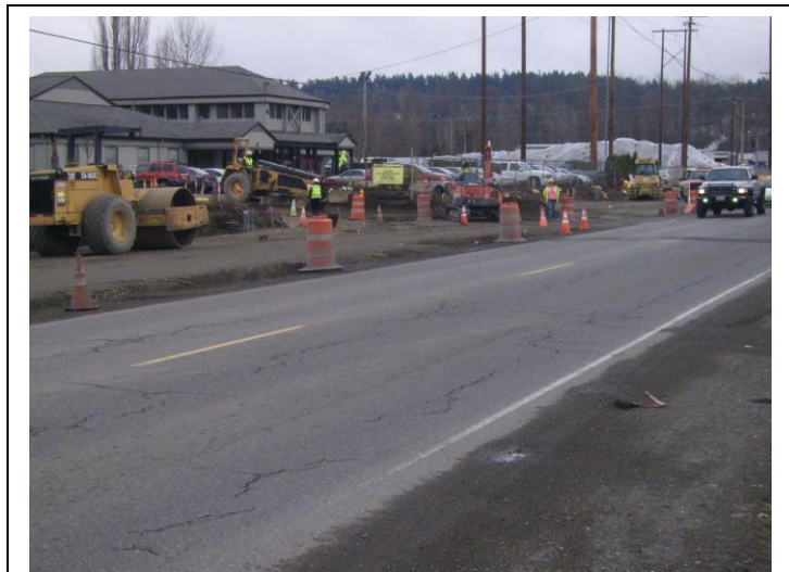
Road Widening of Stewart Road
