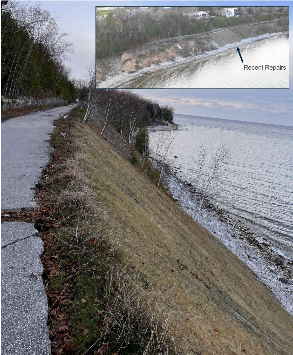
Figure 3.2: Recent Slope Grading and Toe Stone Placement
