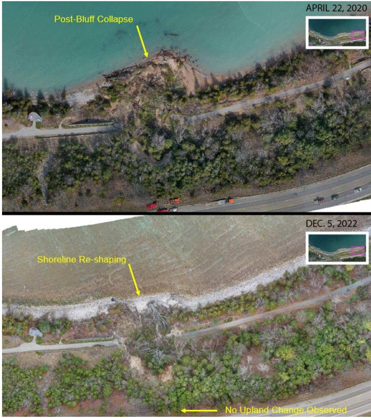
Figure 1.1: Aerial Image Comparison (2020 to 2022) - 2020 Coastal Bluff Collapse
