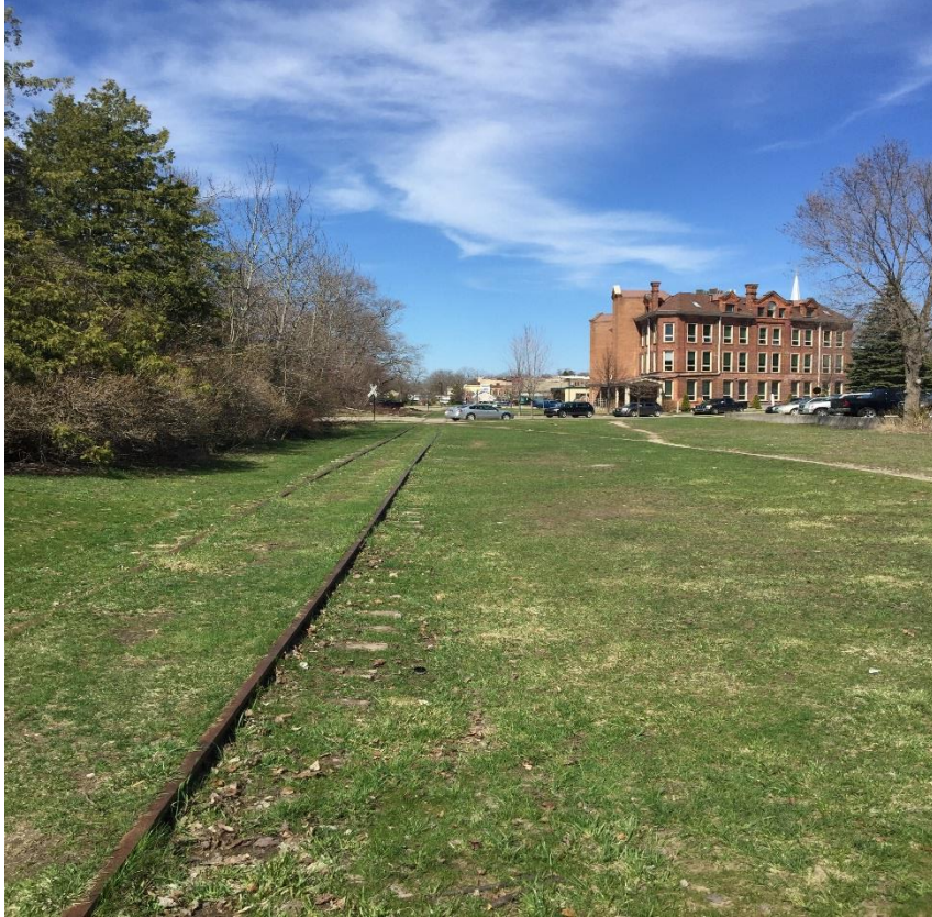
Future location of Phase II of the Downtown Greenway Corridor to be constructed in the summer of 2018
