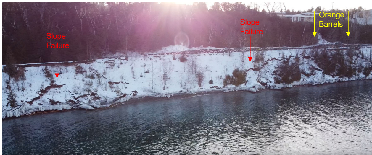
Figure 1: Shoreline Slope Damage (Baird, Dec. 22, 2019)
