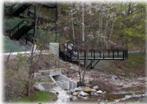
Storm sewer outfall dissipater
