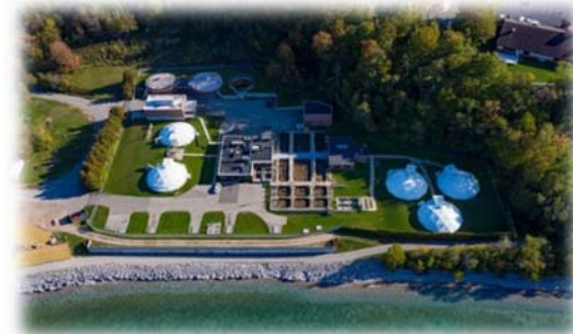
Wastewater Treatment Plant after addition of tank domes
