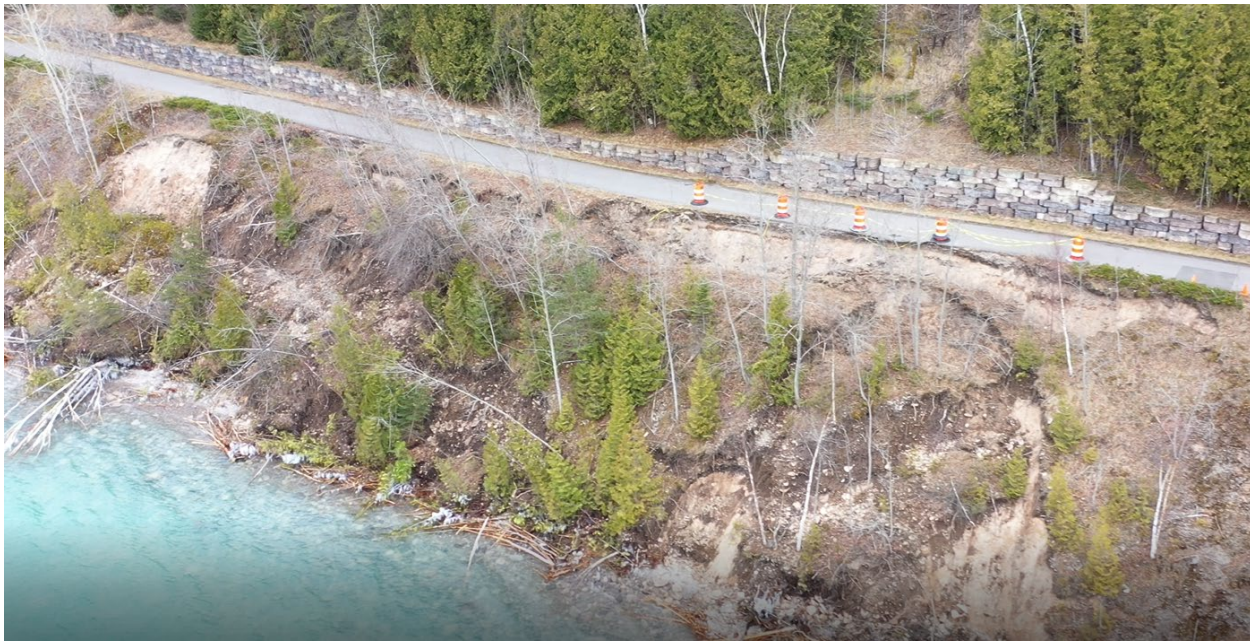
Figure 1.3: Photo 2 – UAV Image of Minor Sloughing Failures (Baird, 2020)
