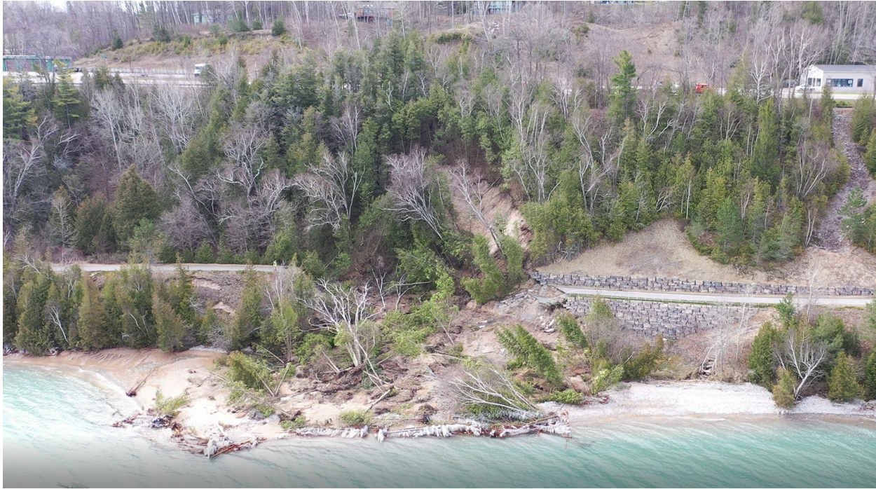
Figure 1.2: Photo 1 - UAV Image of April 13, 2020 Coastal Bluff Slope Collapse (Baird, 2020)
