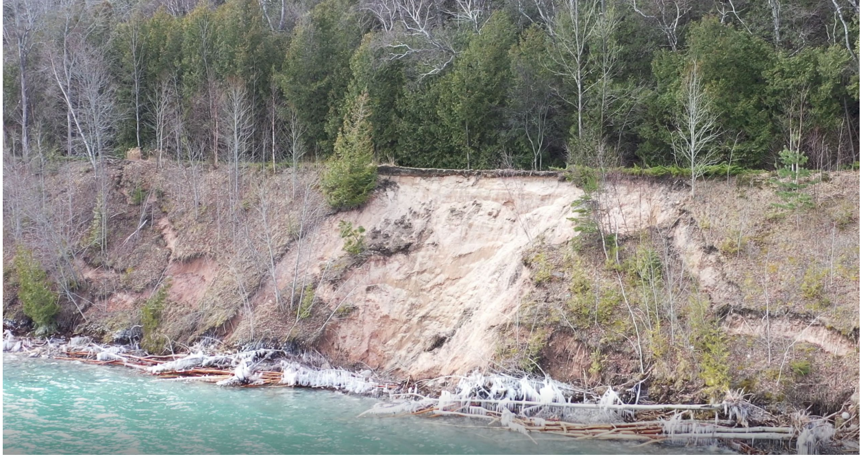
Figure 2.11: Existing Slope Failure and Nearshore Bluff Recession
