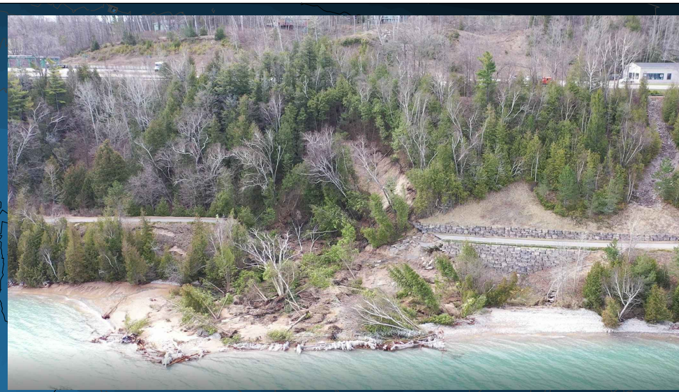
PHOTO 1 APRIL 13, 2020 COASTAL BLUFF COLLAPSE
