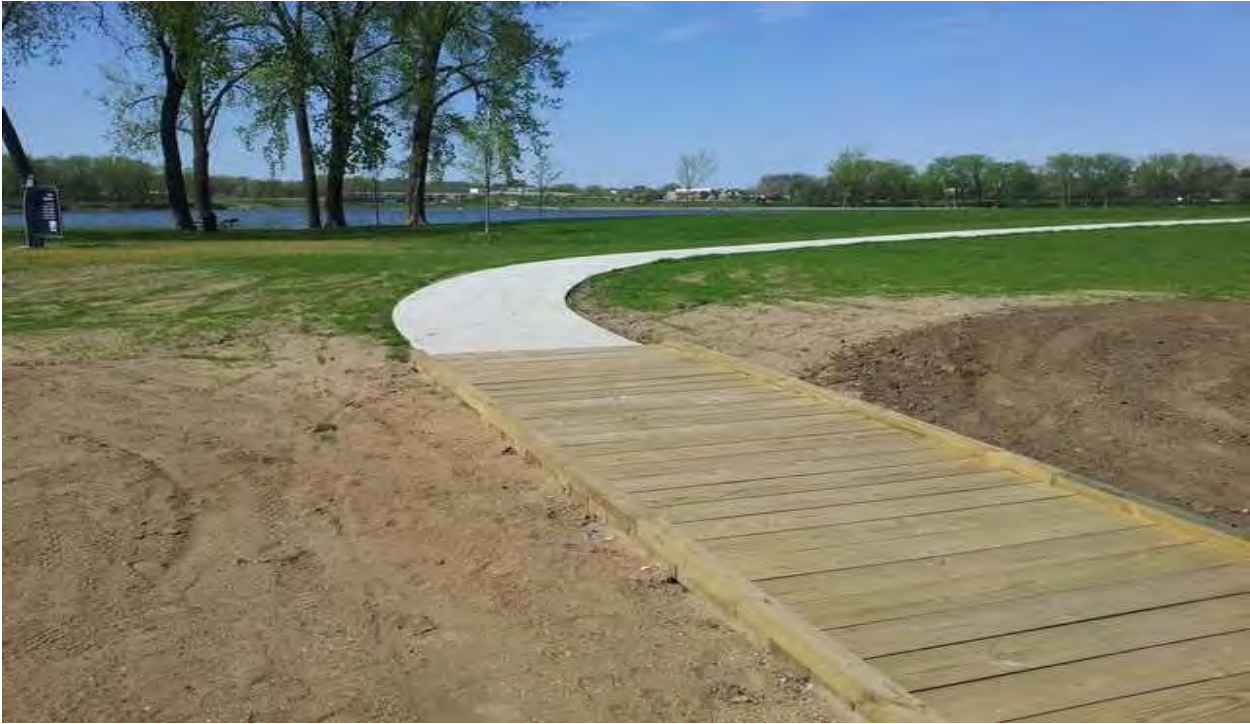
Site-Built Repositionable Boardwalk
