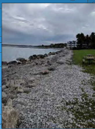
PHOTO 2 FAILING REVETMENT
