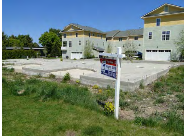
Vacant building pads serve as soil caps, an essential component of the site remedy
