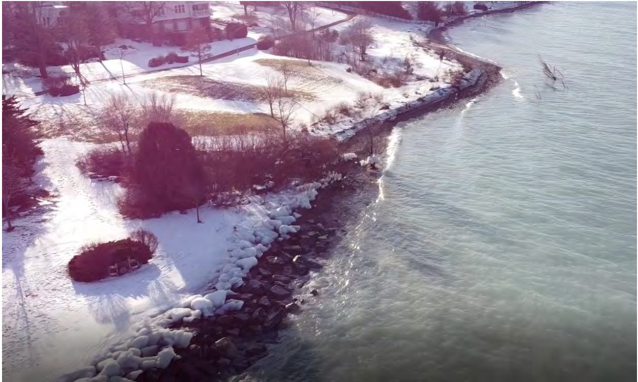
Figure 2.21: Existing Solanus Mission Beach Shoreline – Photo 3 of 4 (Baird, 22 December 2019)
