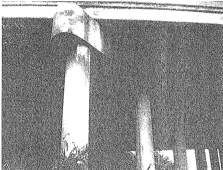
Pier 2W – Leaking and efflorescence on beam ends and pier cap
