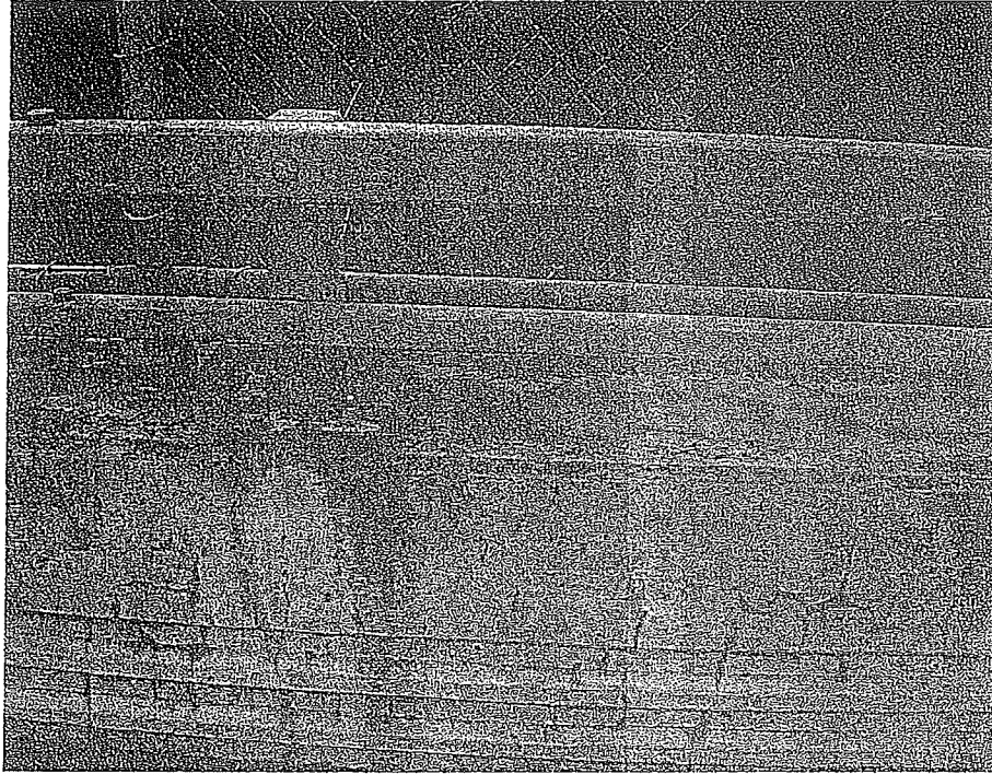
Map cracking in concrete rail
