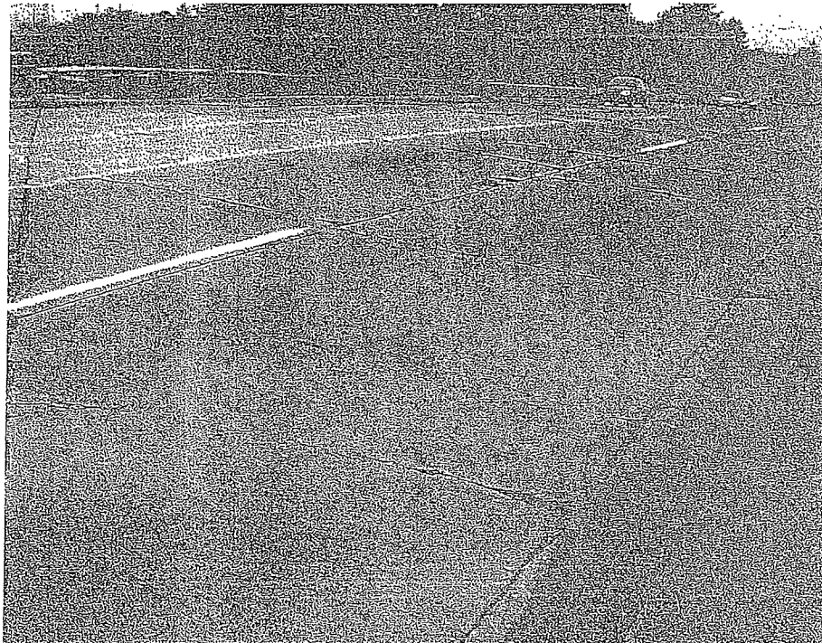
Cracks and spalls in approach slab
