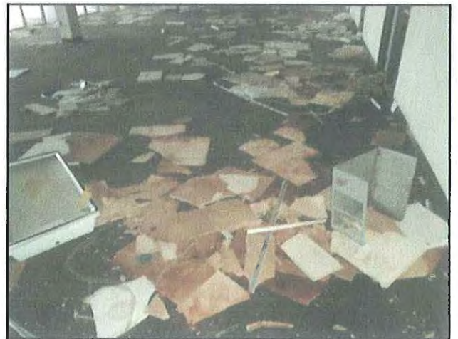
2 : 6th Floor - Water Damage (2)
