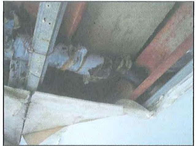
38 : Canopy Water Damage (1)
