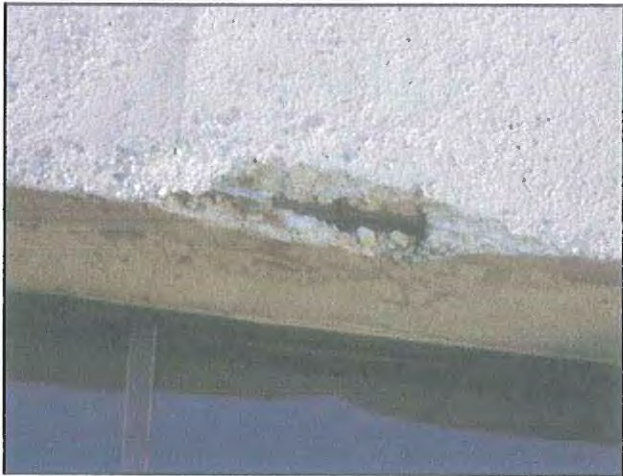
49 : Exterior Exposed Rebar (4)
