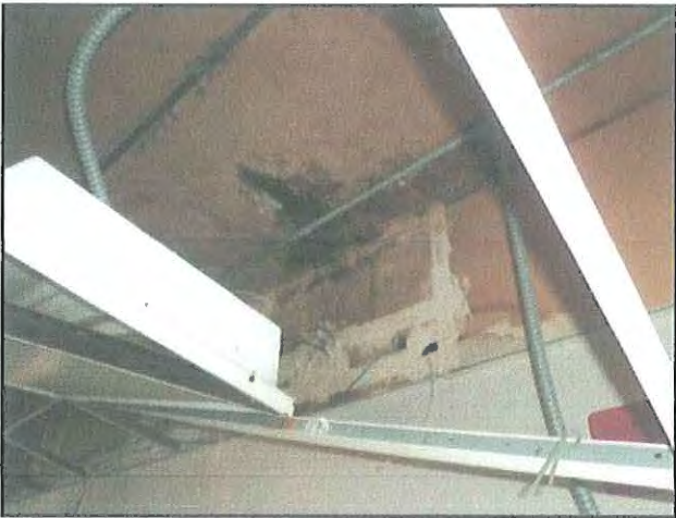
1 : 6th Floor - Water Damage (1)
