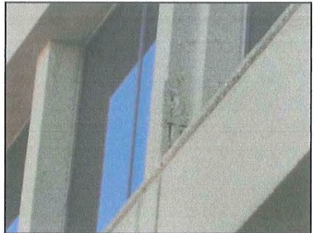
46 : Exterior Exposed Rebar (1)
