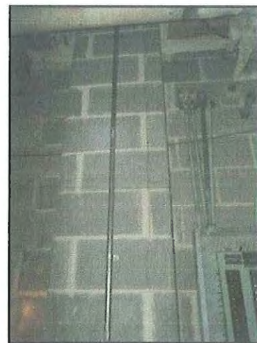
10 : Basement - Block Wall Cracking (1)
