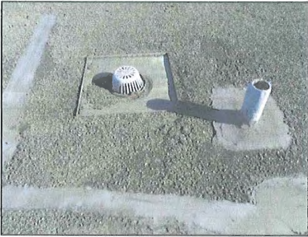
127 : Roof - Drains & Vents (2)
