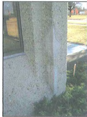
44 : Exterior Cracking & Patching (2)
