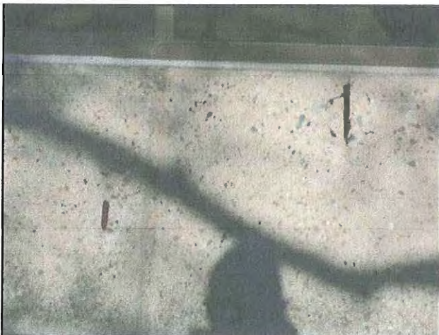
47 : Exterior Exposed Rebar (2)
