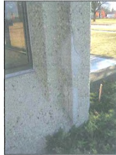
44 : Exterior Cracking & Patching (2)
