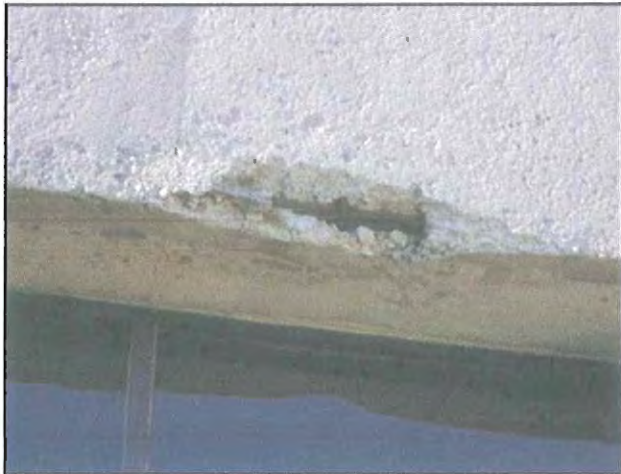
49 : Exterior Exposed Rebar (4)
