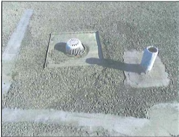
127 : Roof - Drains & Vents (2)
