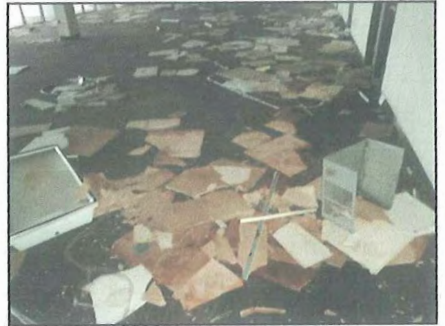
2 : 6th Floor - Water Damage (2)
