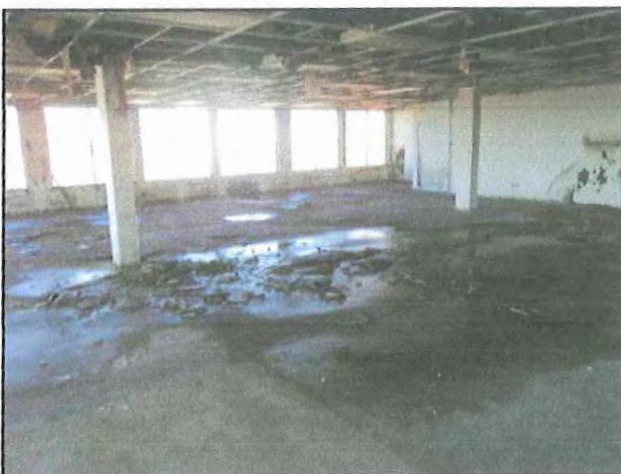
5 : 7th Floor Water Damage (2)
