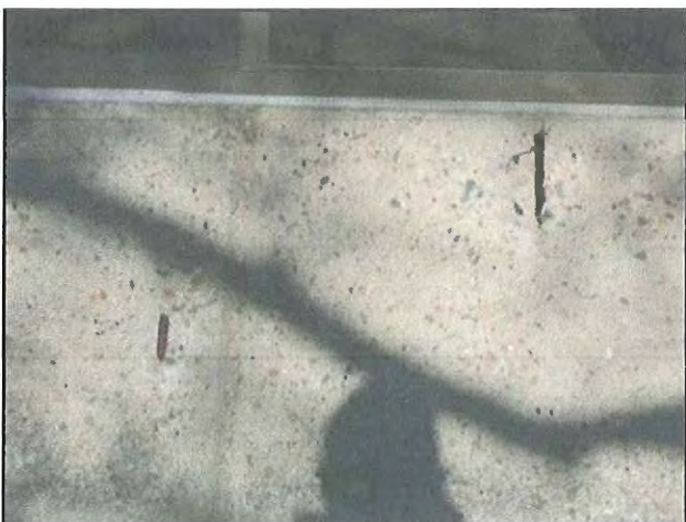
47 : Exterior Exposed Rebar (2)
