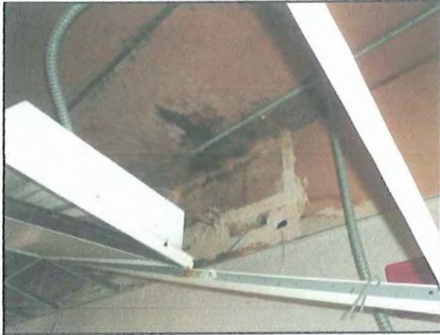
1 : 6th Floor - Water Damage (1)
