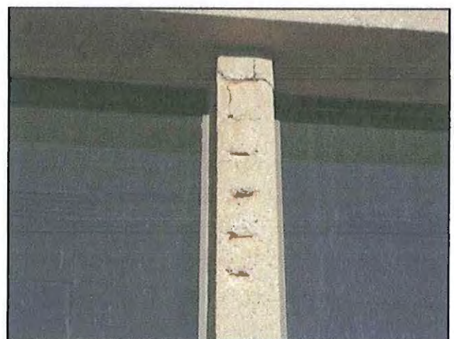
48 : Exterior Exposed Rebar (3)
