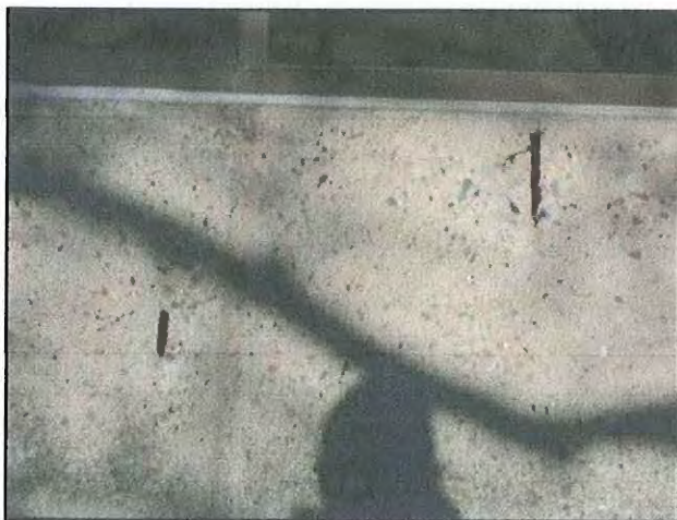
47 : Exterior Exposed Rebar (2)
