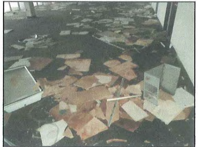
2 : 6th Floor - Water Damage (2)
