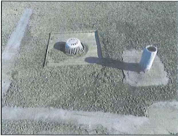
127 : Roof - Drains & Vents (2)
