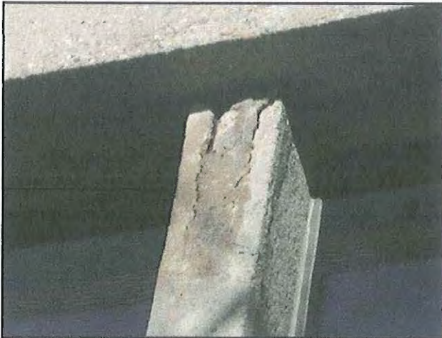
45 : Exterior Cracking & Patching (3)
