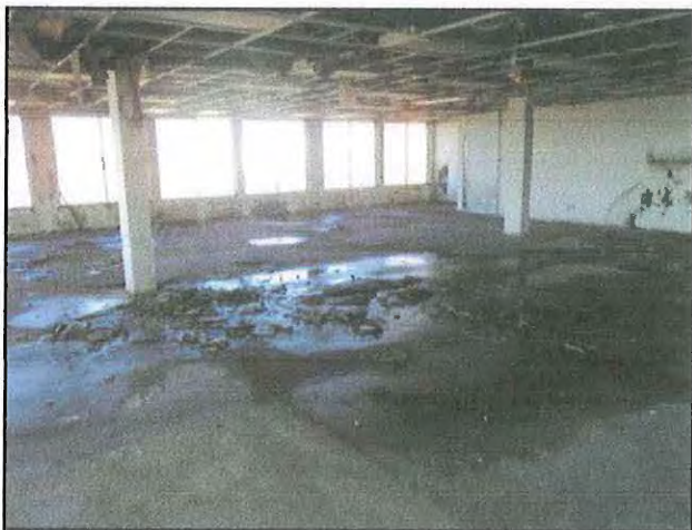
5 : 7th Floor Water Damage (2)
