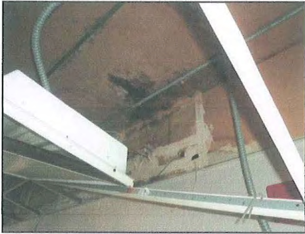
1 : 6th Floor - Water Damage (1)
