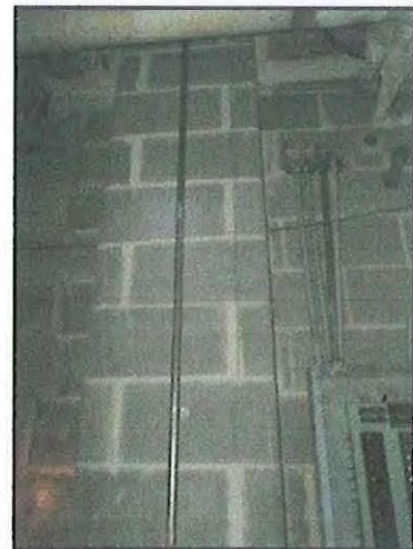
10 : Basement - Block Wall Cracking (1)
