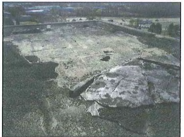
124 : Roof - Damage (1)
