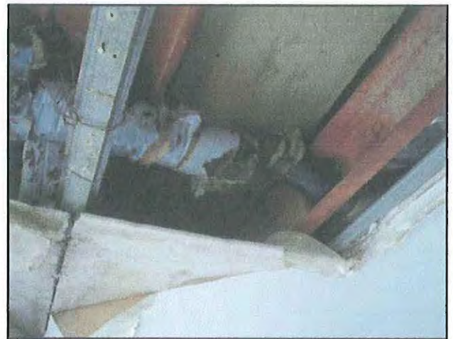
38 : Canopy Water Damage (1)
