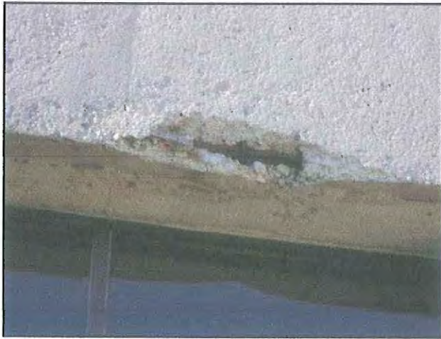
49 : Exterior Exposed Rebar (4)
