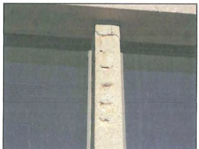
48 : Exterior Exposed Rebar (3)
