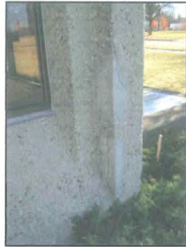
44 : Exterior Cracking & Patching (2)
