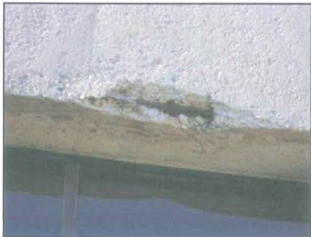
49 : Exterior Exposed Rebar (4)
