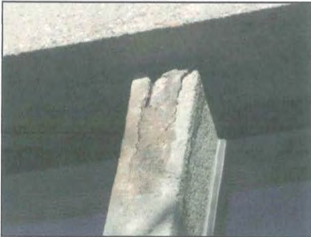
45 : Exterior Cracking & Patching (3)
