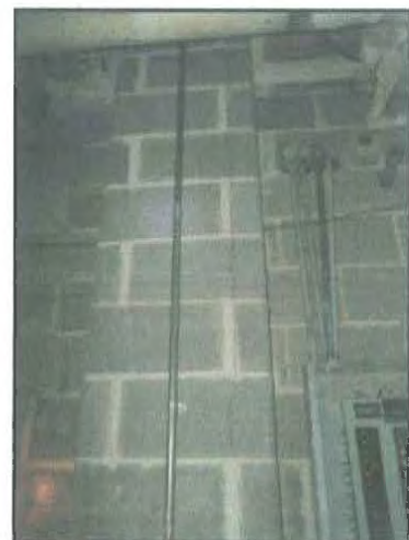
10 : Basement - Block Wall Cracking (1)
