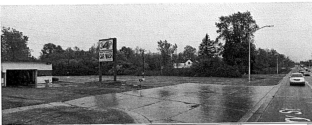
Figure 5 – photo of site from the Car Wash
