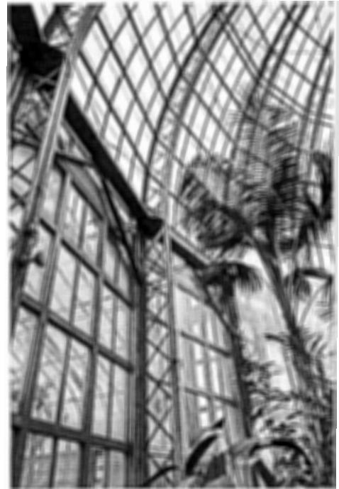
Picture 2: Original truss column in the Palm House
