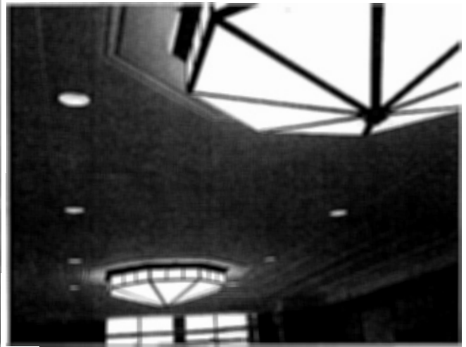
Photo 6: New custom light fixtures in Library.
