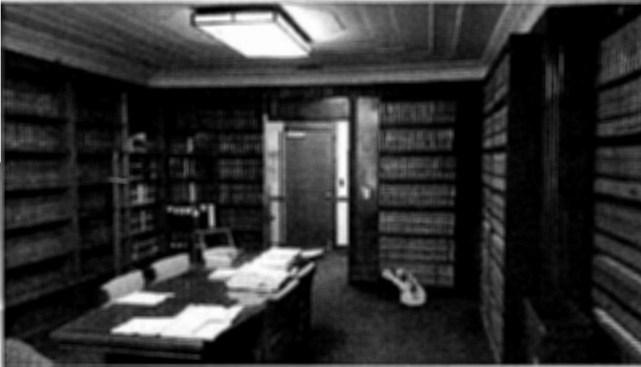
Photo 3: Library prior to restoration with bookcases attached to original wood Panels and surface mounted fluorescent lights.
