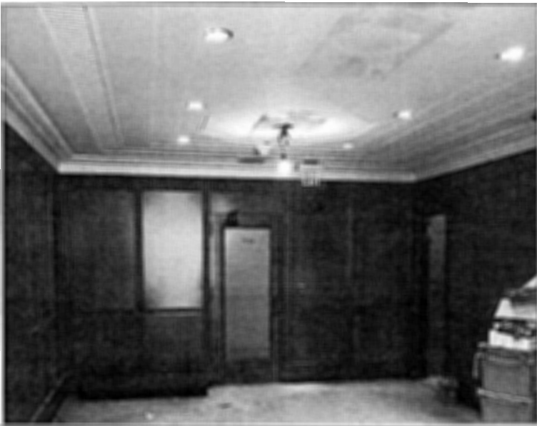
Photo 5: Walnut wall panels restored in the Library.
