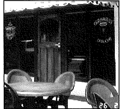
Rehabilitated storefront with incompatible stained glass door.
