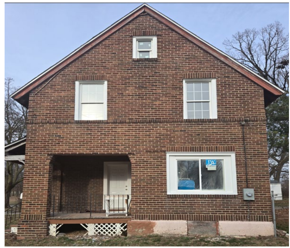
Figure 4: WEST FAÇADE Applicant installed second and third story vinyl windows and the metal door. The vinyl window on the first floor was installed by a previous owner.
