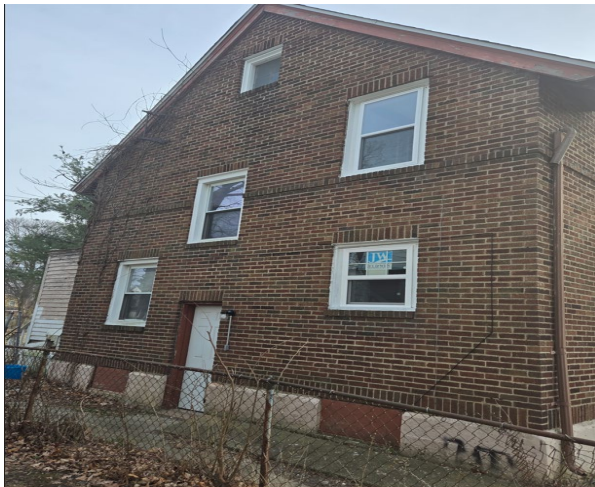
Figure 5: EAST FAÇADE Applicant installed the metal door and installed the vinyl window to the right of the door. The applicant is proposing a new 3 rd story vinyl window. The remaining windows were installed by a previous owner without HDC approval.
