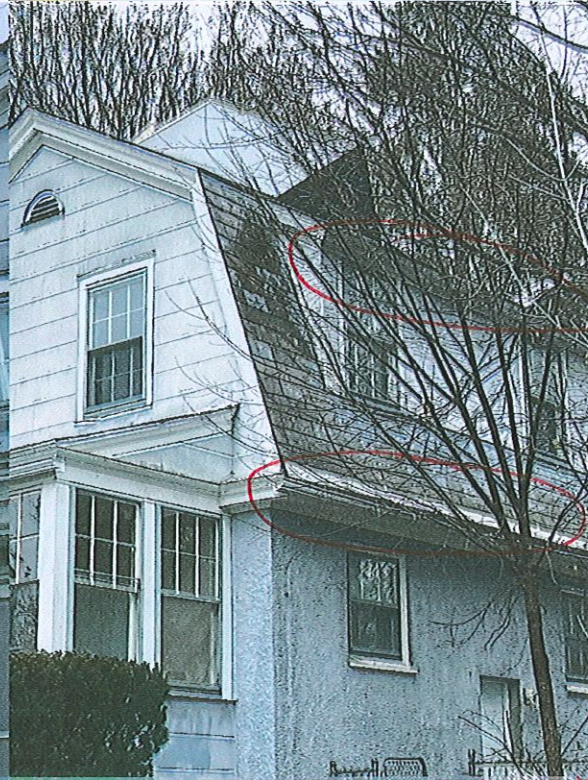
Exposed metal flashing & rotted/missing fascia
