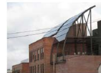
Saranac Building: Consider how a project can take advantage of green technology effective in Spokane’s climate.
