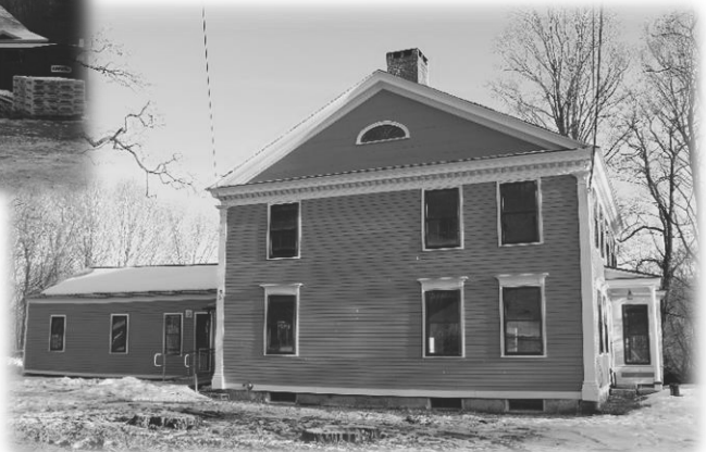
Windham & Windsor Housing - Noyes House Restoration
