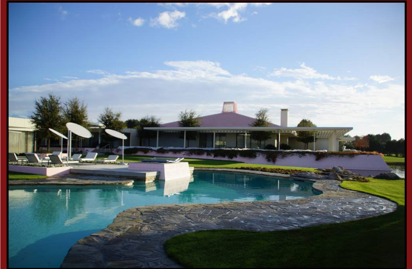
Sunnyslands (1966), designed by architect A. Quincy Jones.
