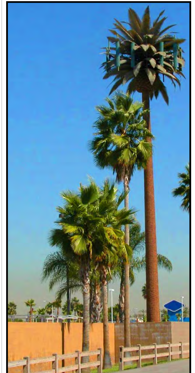
Palm tree cell tower concealment.
