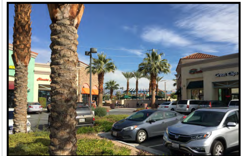
Parking arcades with shade and spaces close to shops.
