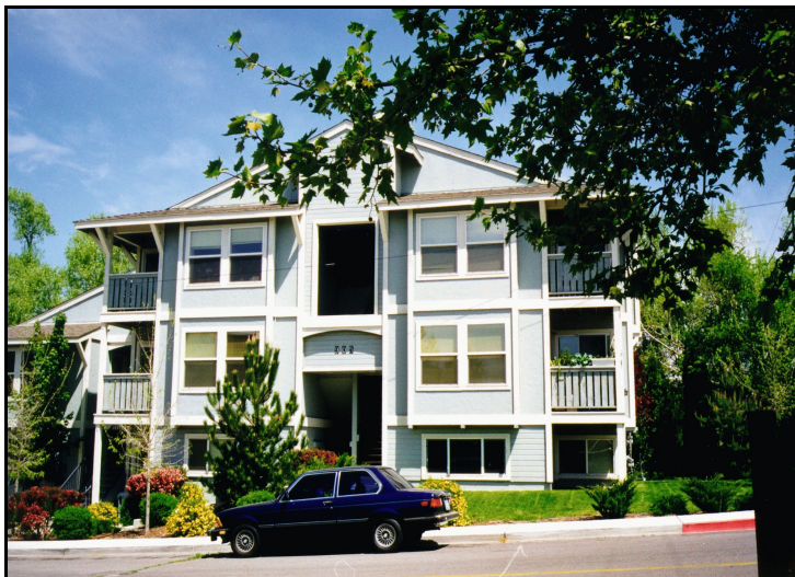
An example of significant wall articulation
