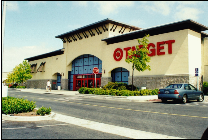
Large buildings can be appropriately designed and detailed to create a quality appearance
