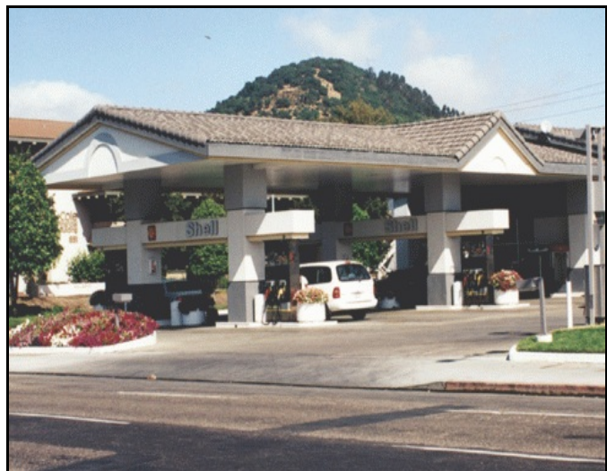
The roof lines and materials used in this service station canopy are appropriate
