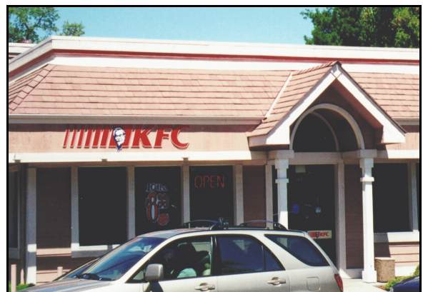
An entry element, wood siding, window trim, and wood-look roofing materials help this building to look less like a 'franchise' use
