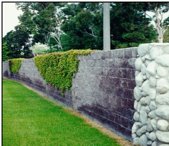
A wall that features appropriate materials and vines
