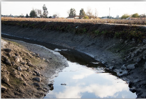
Figure 1: Channels, Streams, and drainage are impacted by increased upstream impervious surface
