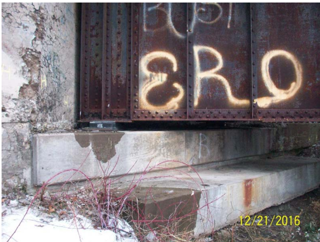
Photo 4 – Abutment seat and jacking pad, looking south
