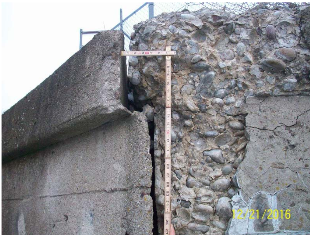
Photo 8 – Close-up of separation at north wingwall construction joint
