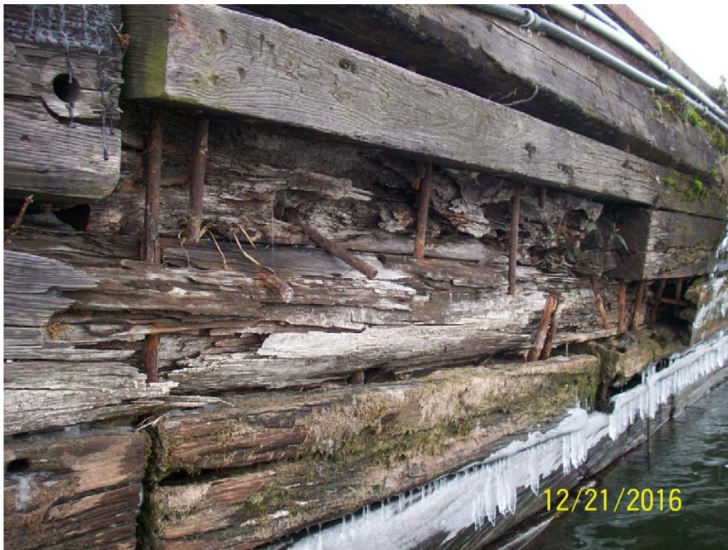
Photo 12 - Timber cribbing wall, close-up of decay near STA 140
