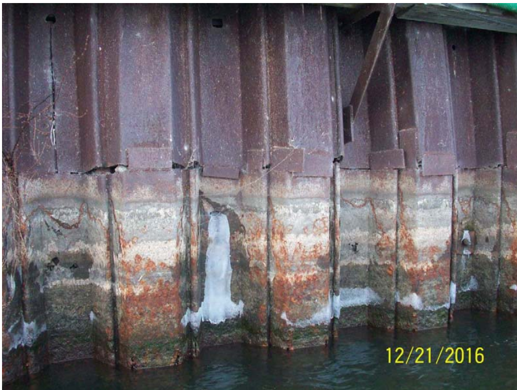
Photo 26 - Sheet pile wall, irregular welded splices at STA 750
