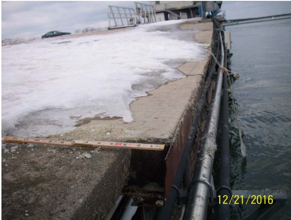
Photo 15 - Top of timber cribbing wall, showing concrete slab displacement at STA 304
