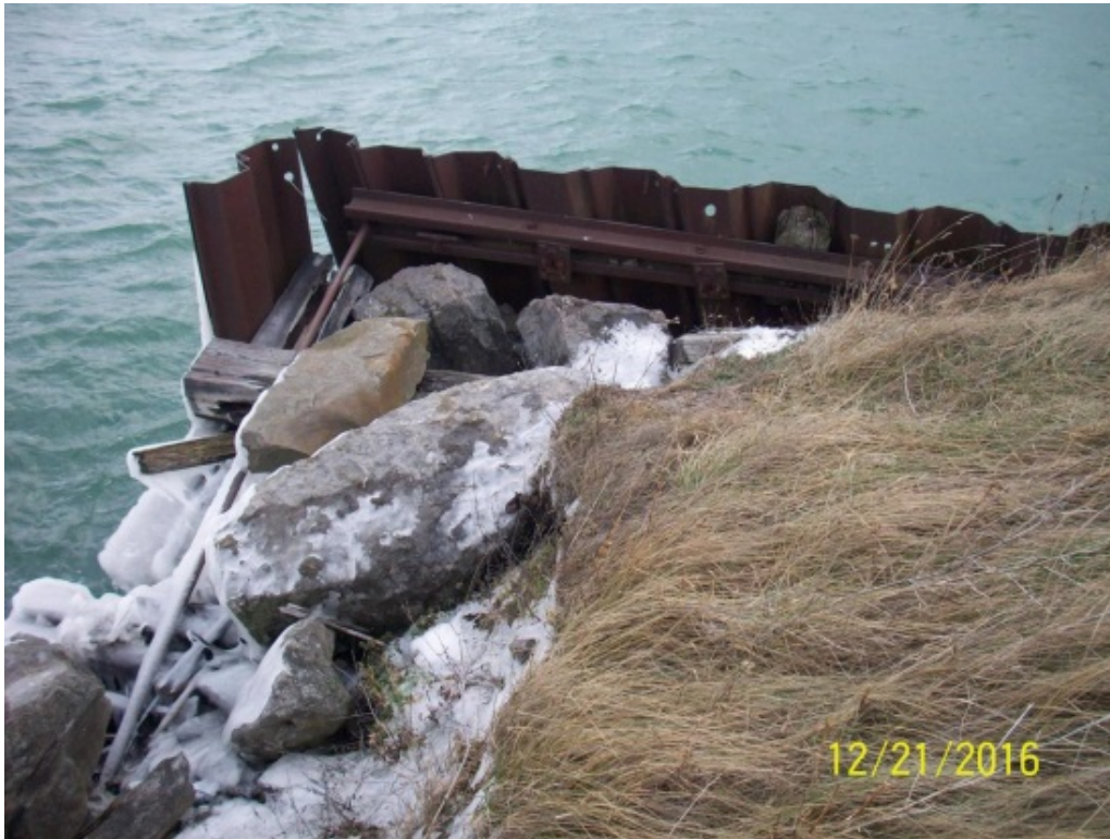
Photo 31 – End of sheet pile wall at northwest corner of pier,
