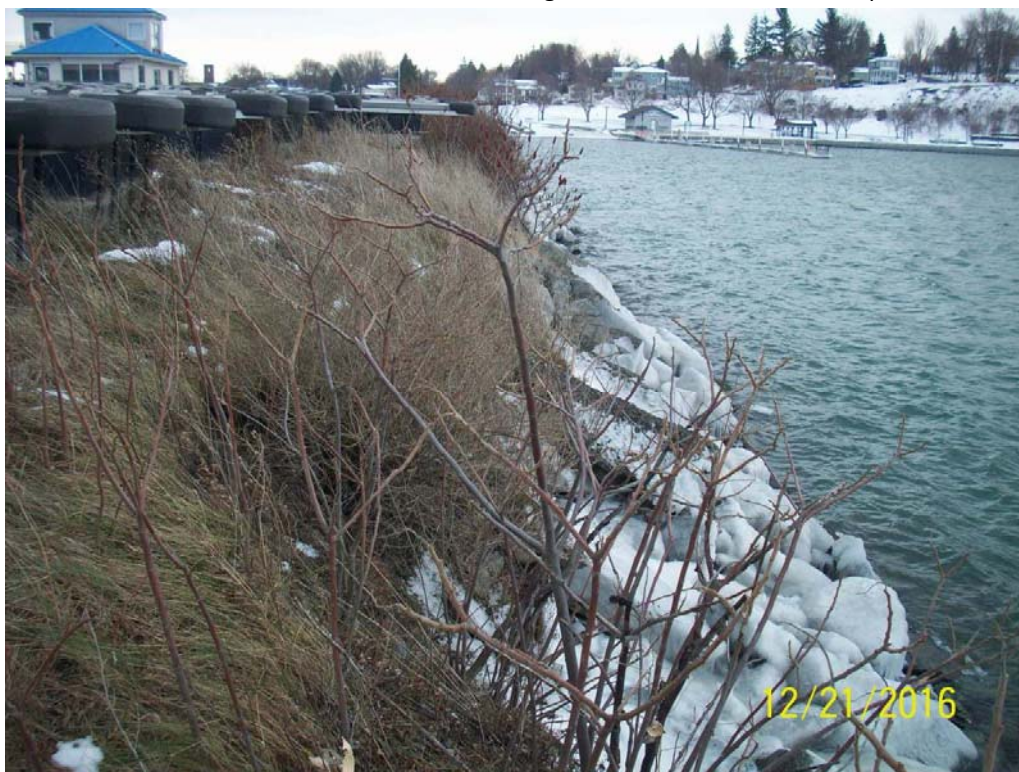
Photo 40 – Stone bank protection at west side of pier
