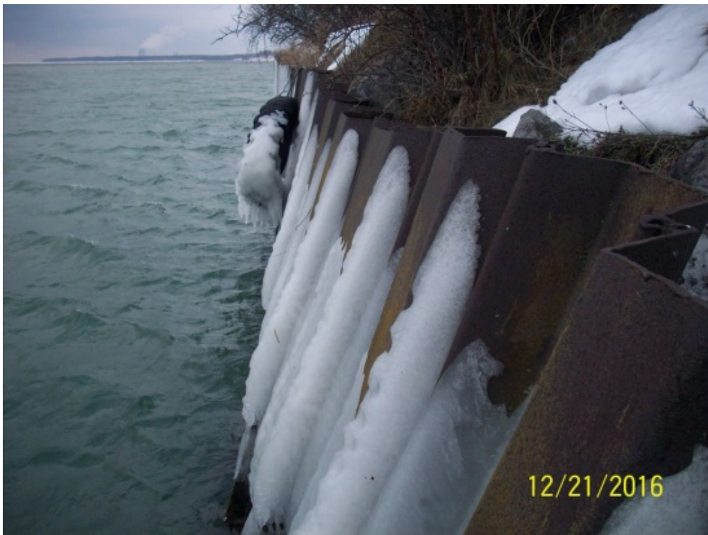
Photo 32 – Leaning sheet piles at northwest corner of pier
