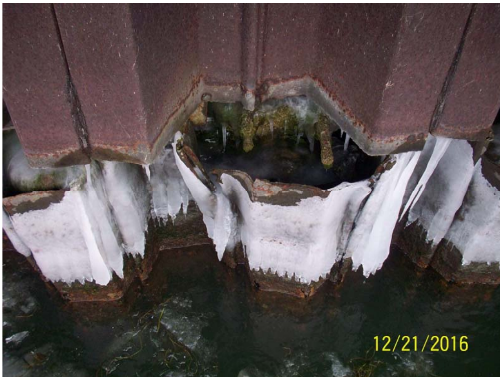
Photo 28 - Sheet pile wall, mis-matched pile "splice" near STA 800
