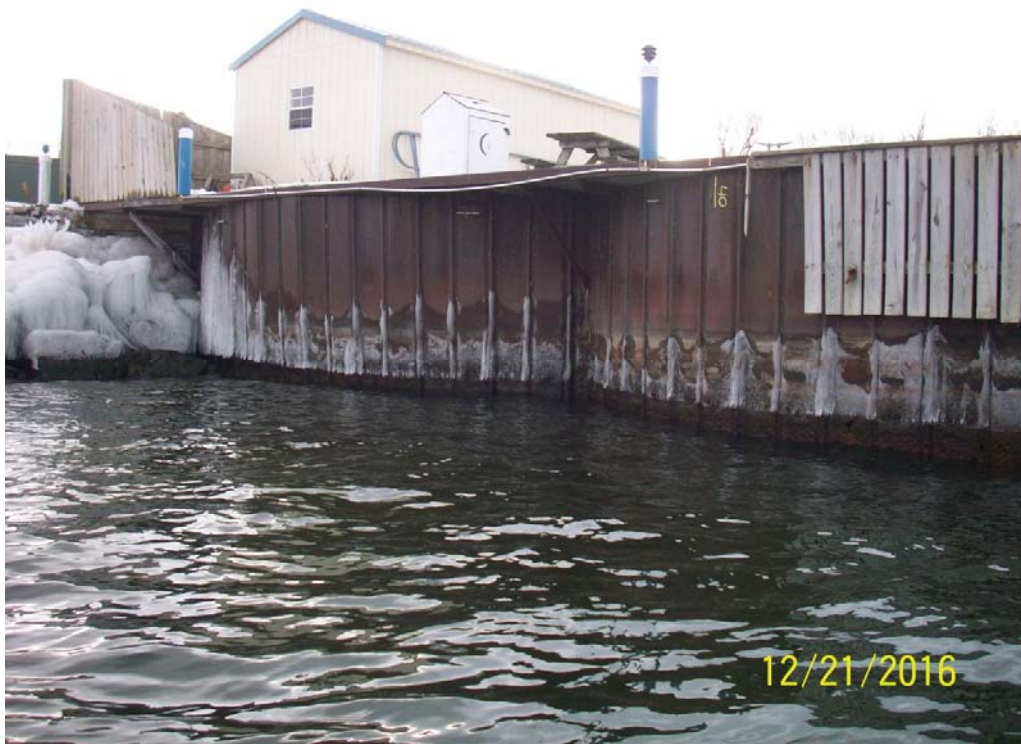
Photo 3 – Cellular sheet pile wall near STA 40
