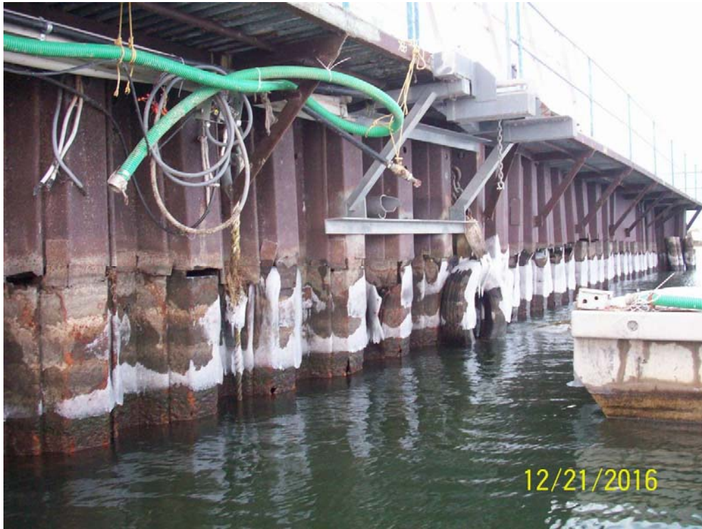
Photo 27 – Sheet pile wall, irregular welded splices near STA 780
