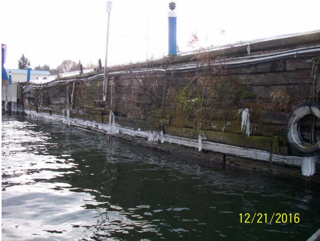
Photo 9 – Timber cribbing wall, looking south near STA 200
