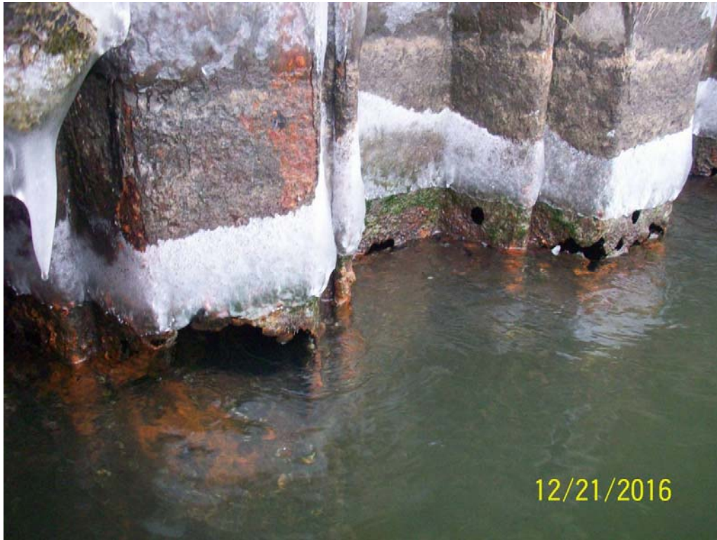
Photo 21 – Sheet pile wall, close-up of typical holes near low water level at STA 350
