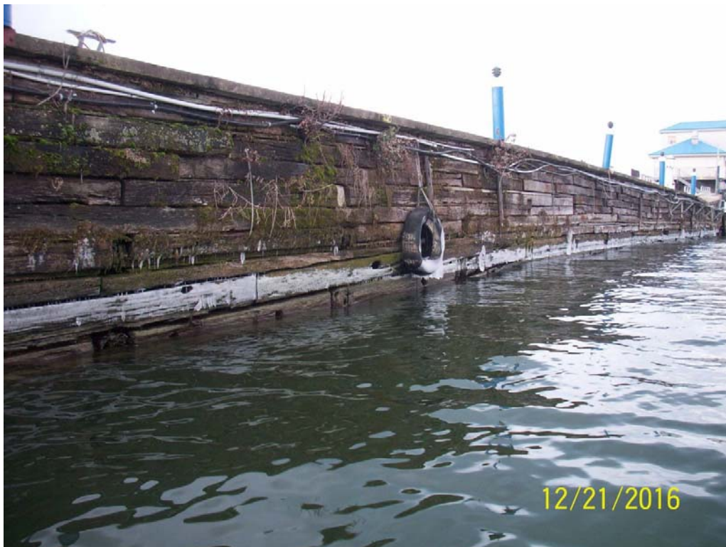
Photo 10 - Timber cribbing wall, looking north near STA 200
