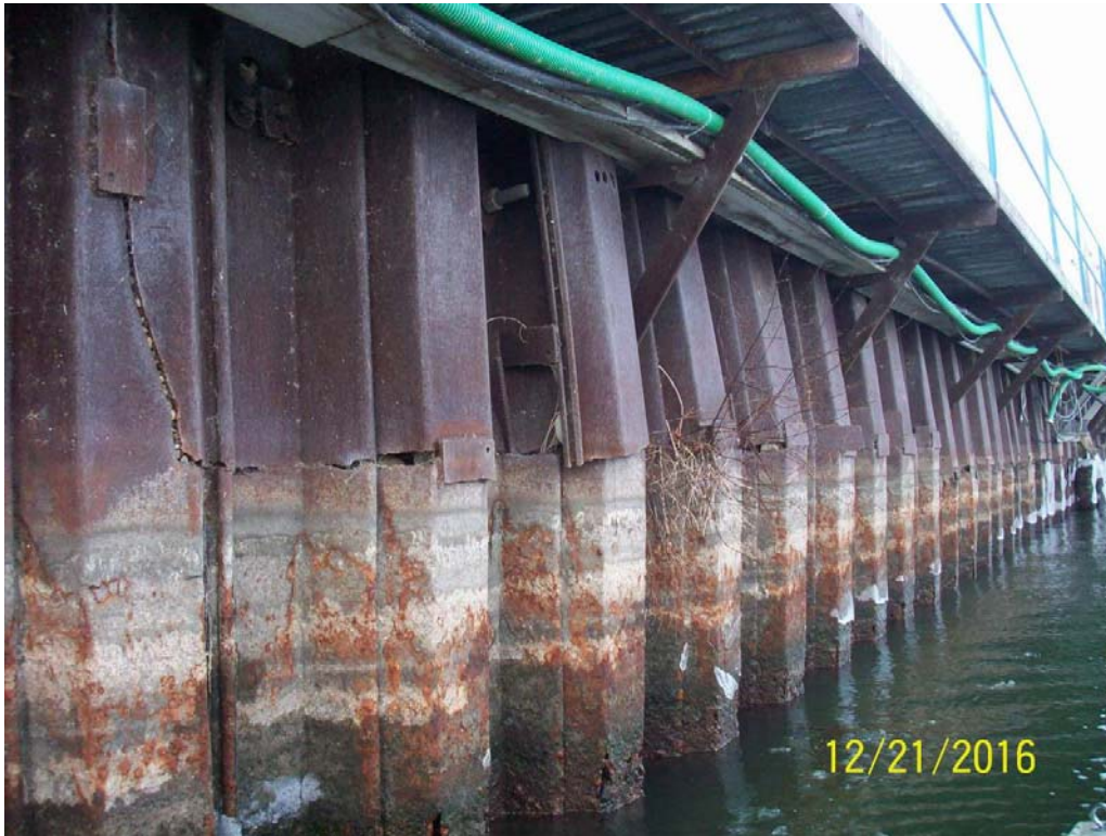
Photo 25 - Sheet pile wall, irregular welded splices beginning at STA 730
