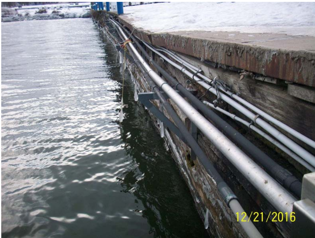
Photo 14 - Top of timber cribbing wall, showing settlement between STA 300 and 344
