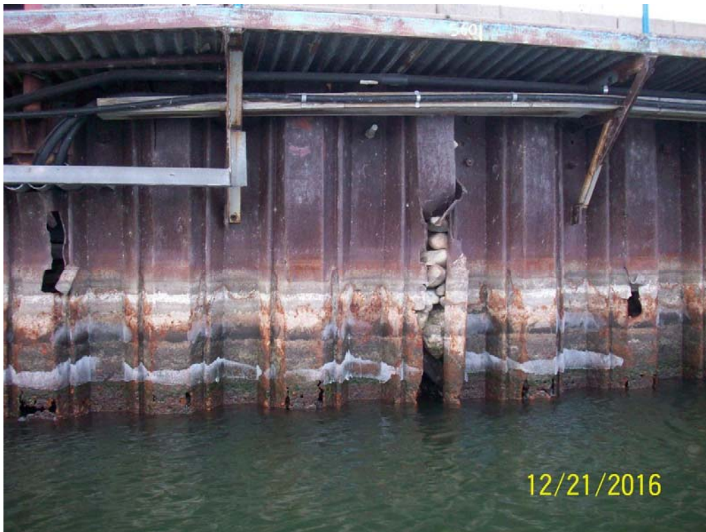
Photo 24 - Sheet pile wall, torn piles near at STA 560
