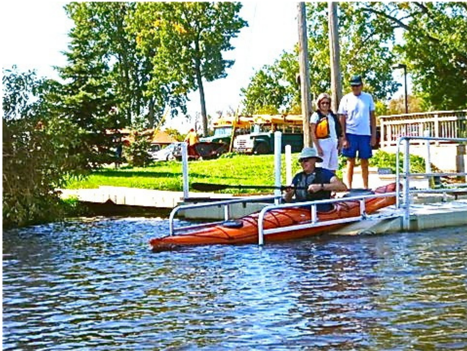
New handy cap loading ramp - Dexter (on rollers)
